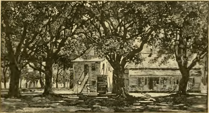
Pakenham's Headquarters (from the rear).
