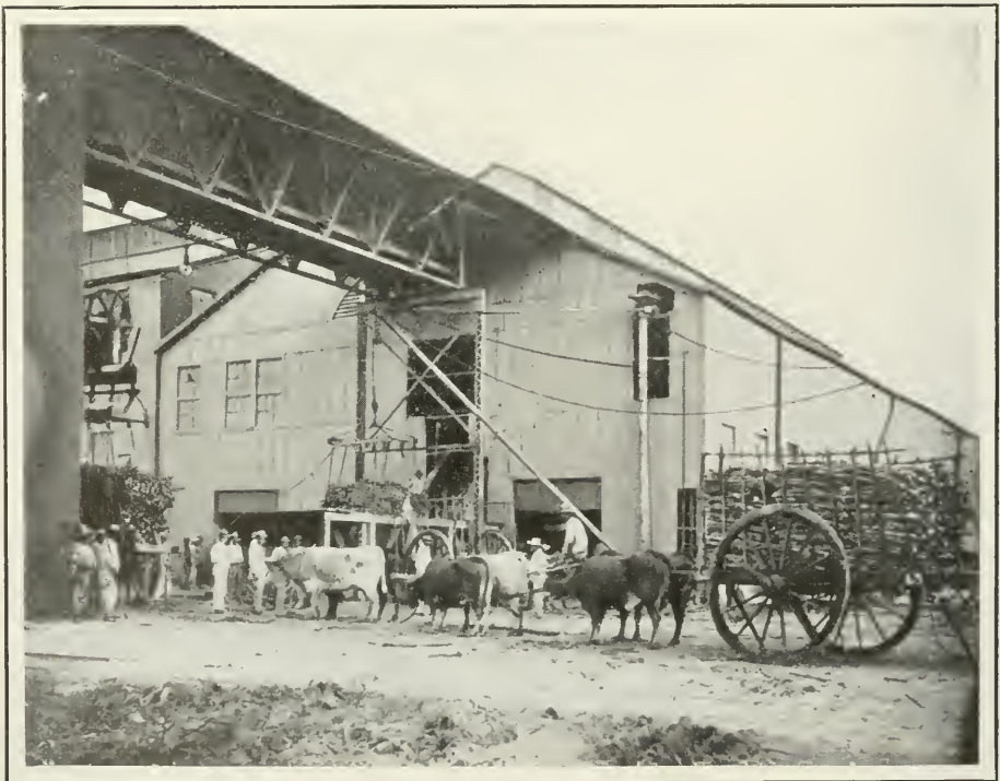
The cane after being cut and stripped of its leaves is brought to the mill in great carts. The crane takes up the contents of the carts at one lift.
