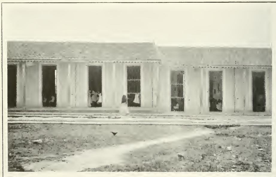
View of Cottages
