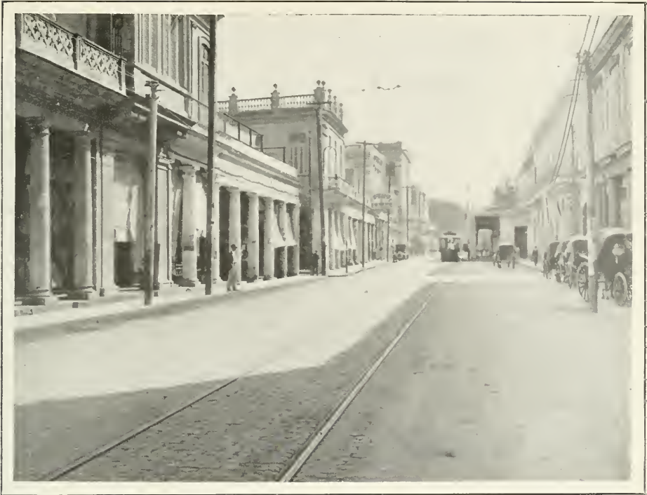
New Pavement Havana Streets.
