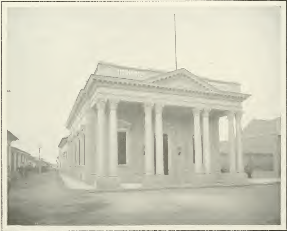
New Bank Building at Camaguey
