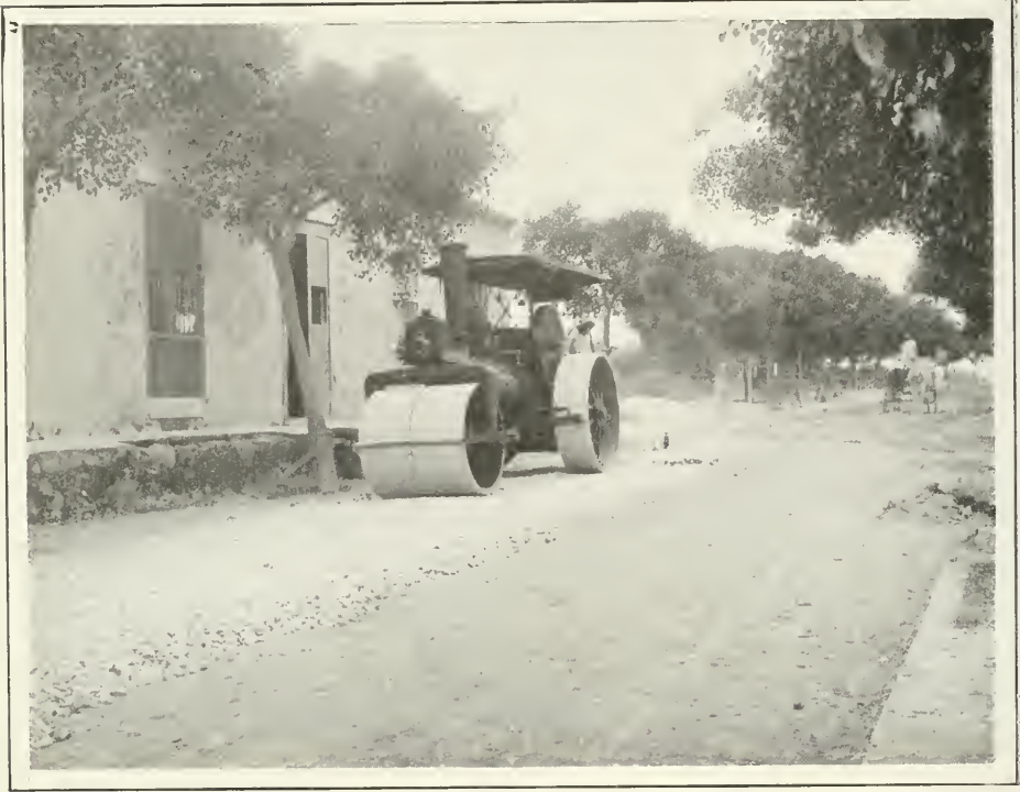
Working on Macadam Road to Cemetery, near Havana.
