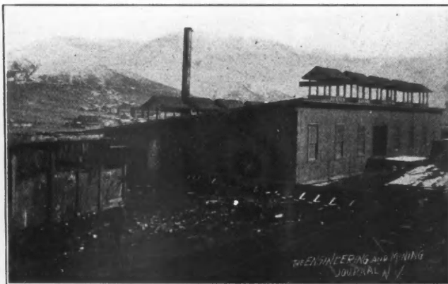
BOSTON & MONTANA SETTLING TANK AND CLEAN-UP HOUSE
