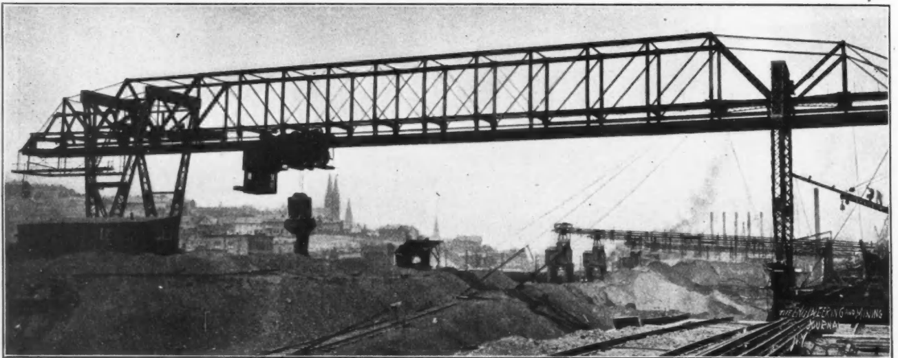
GENERAL VIEW OF ORE-HANDLING BRIDGE AT CARNEGIE STEEL COMPANY'S PLANT, DUQUESNE, PENN.
