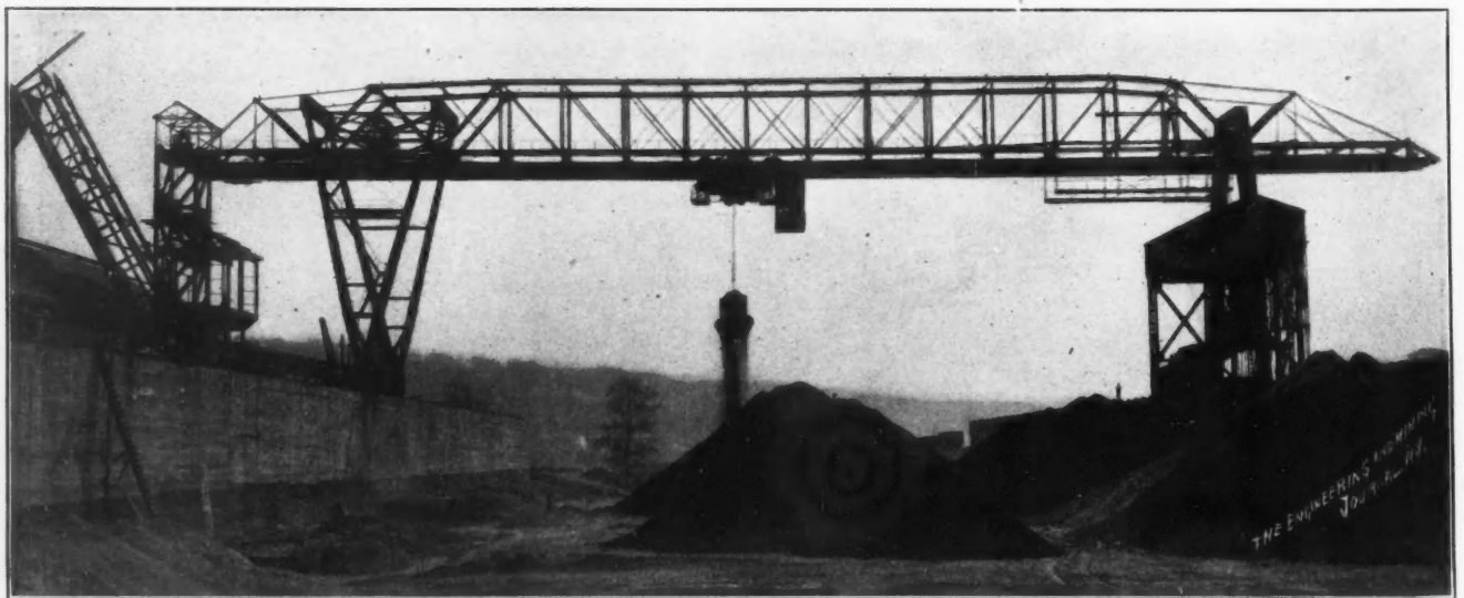
HANDLING ORE AT YOUNGSTOWN, OHIO, WITH A HEYL & PATTERSON BRIDGE
