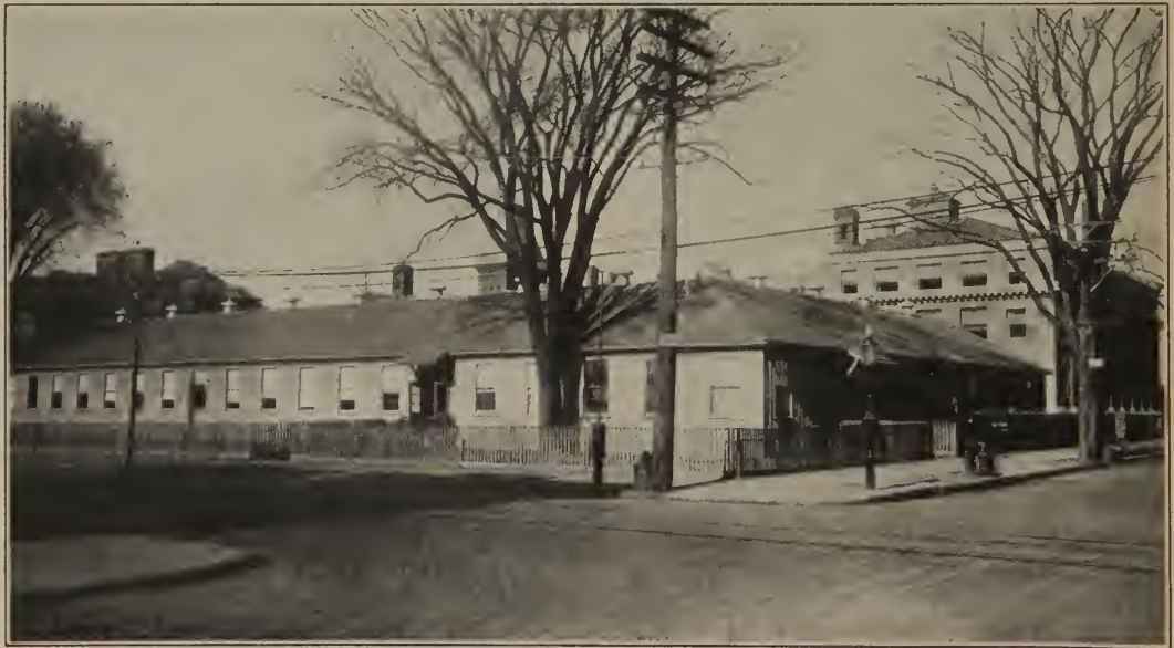
BARRACK, BRADY LABORATORY ANNEX
