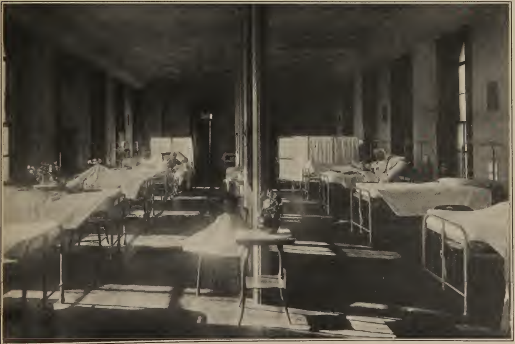
INTERIOR OF EAST WARDS PRIOR TO REHABILITATION
