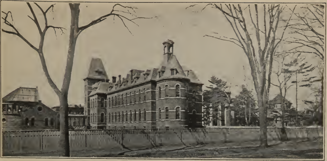
FAÇADE OF EAST WARDS PRIOR TO REHABILITATION WITH FARNAM OPERATING SUITE TO THE LEFT
