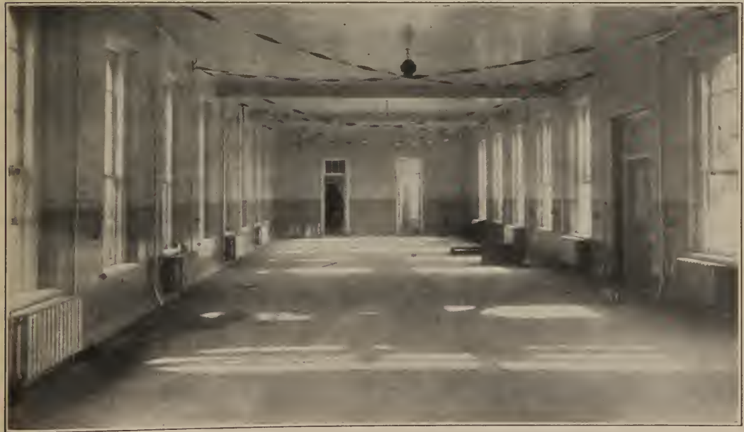
EAST WARDS, EXTERIOR AND INTERIOR VIEWS, AFTER REHABILITATION
