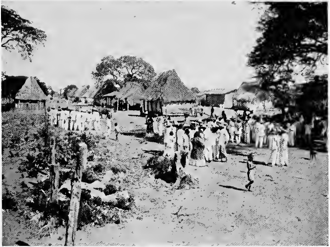
A station of the "Pan-American" south of Tehuantepec
