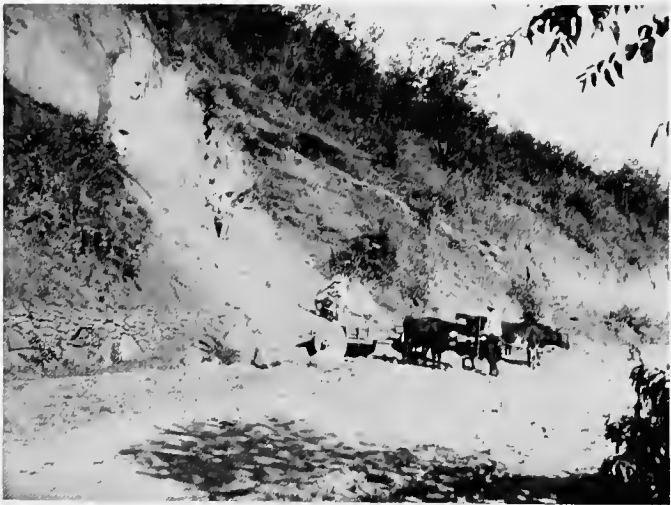
Repairing the highway from Tegucigalpa to the coast
