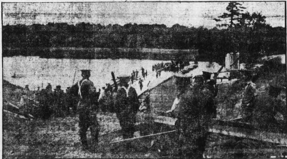
Constructing an Artillery Pontoon Bridge over the Jacques Cartier River. —Courtesy of Canadian Northern Ry.
