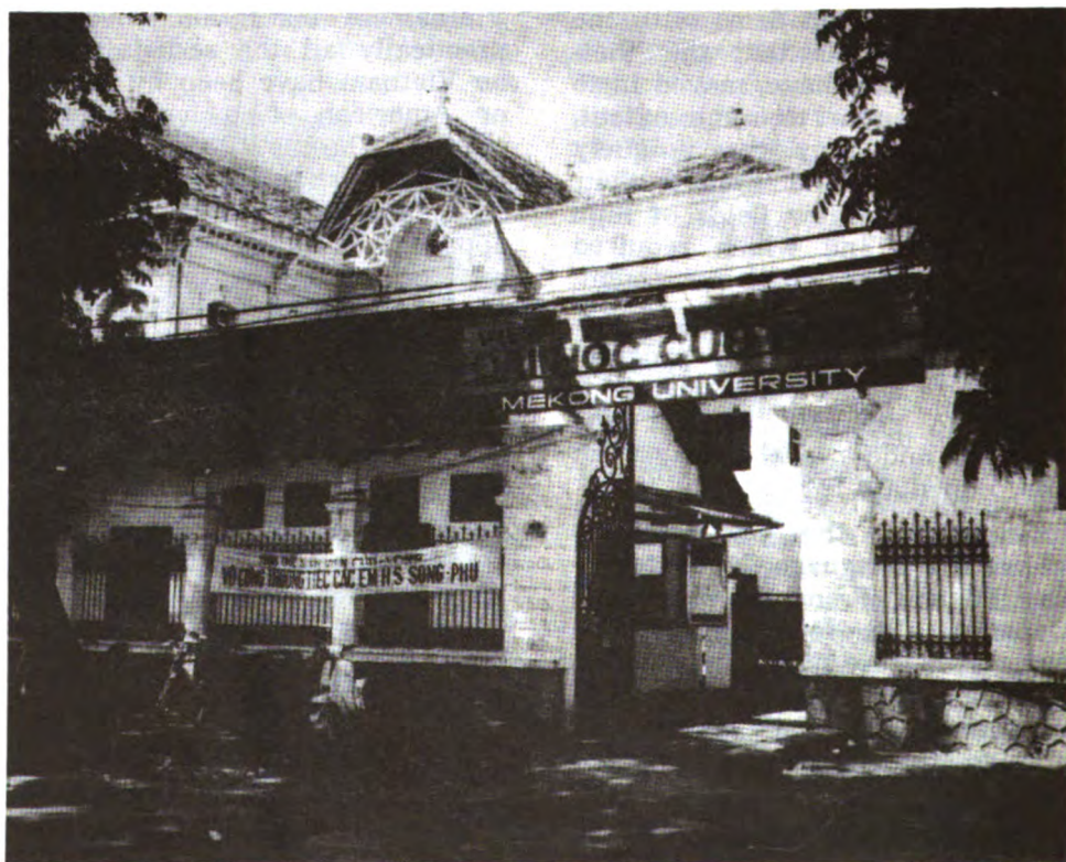
Renovated Army Bachelor Officers' quarters houses Mekong University.
