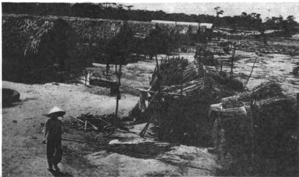
Temporary houses for refugees being built with COREV assistance.
