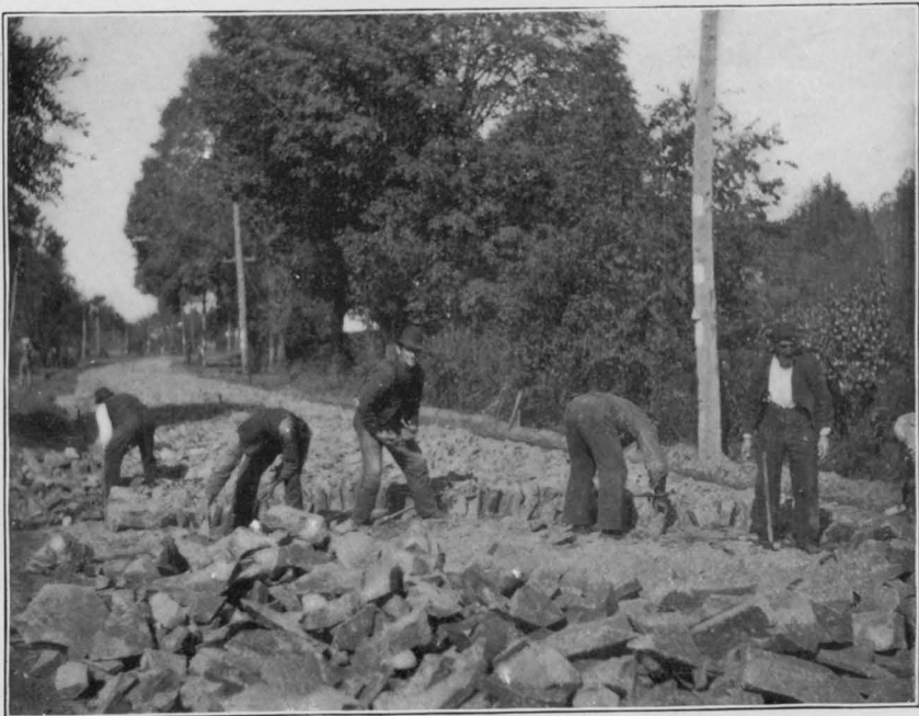
FIG. 2.—STATE ROAD IN MASSACHUSETTS. (LAYING THE TELFORD FOUNDATION.)
