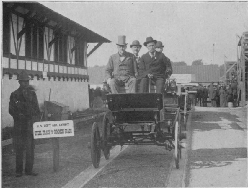
FIG. 1.—HORSELESS CARRIAGE PROPELLED BY ELECTRICITY ON STEEL-TRACK WAGON ROAD.
