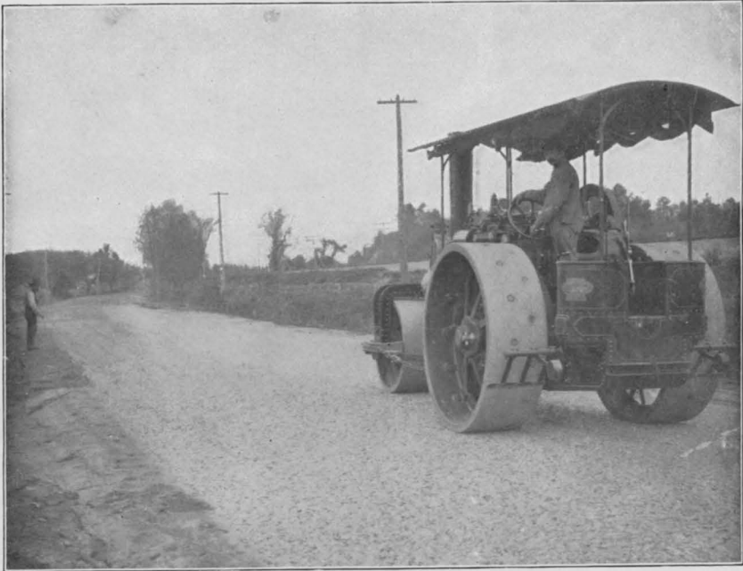
FIG. 1.—SURFACING A MACADAM ROAD IN MASSACHUSETTS.
