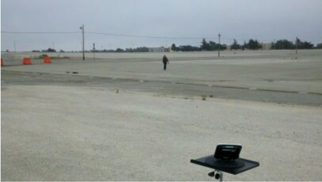
Figure 42. Measuring Out the Test Range
