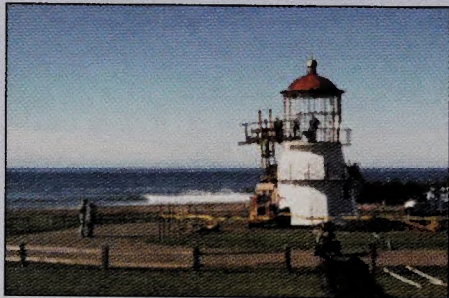
Cape Mendocino Lighthouse restoration at Mal Coombs Park, Shelter Cove, in 2000.
