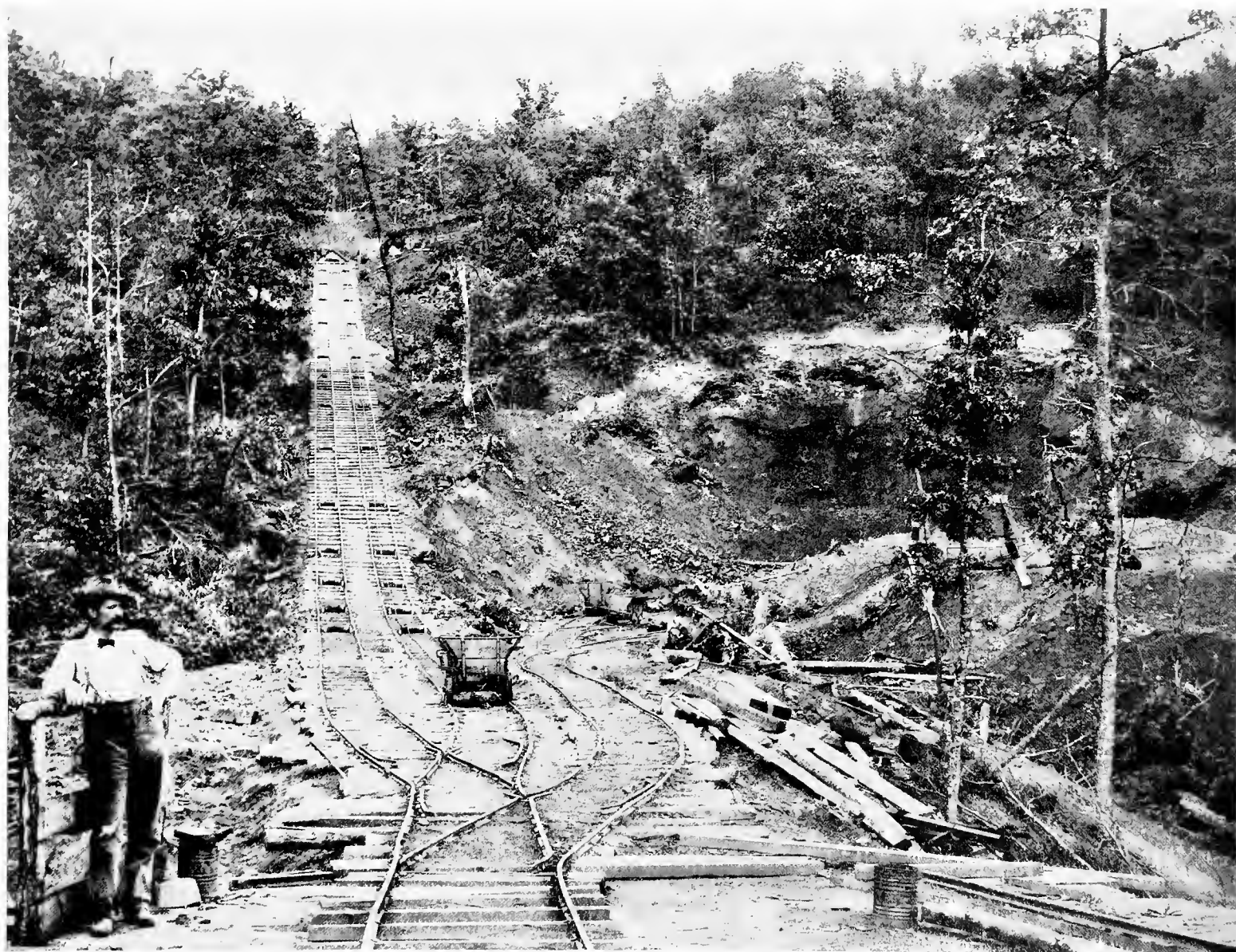
HUDDLESTON MINE, POTTS VALLEY, VA., SHOWING INCLINE. (Ore used at Victoria Furnace.)
