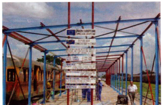
Building site overhead shelter
