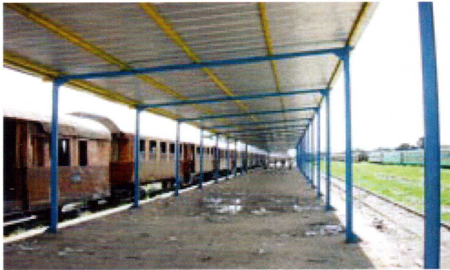
Finished overhead shelter
