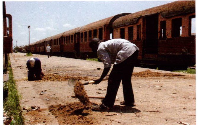
Preparation of the building site overhead shelter
