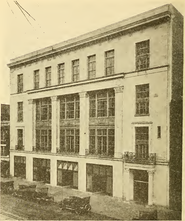
1310 TO 1320 G STREET NORTHWEST
