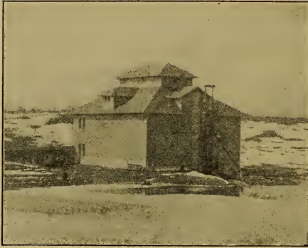
Fig. 79.—LOCAL COLD STORAGE
