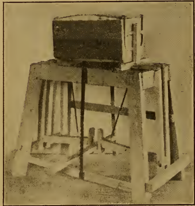
Fig. 71.—A HOME-MADE BOX NAILING PRESS
