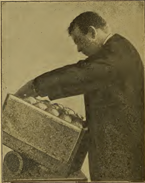
Fig. 134.—TESTING FOR END PLAY
