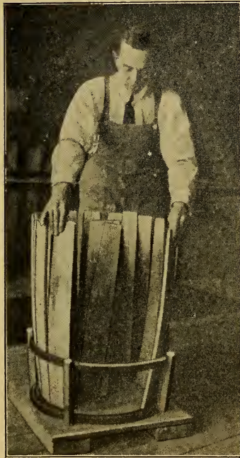
Fig. 38.—FORM FOR SETTING UP A BARREL
