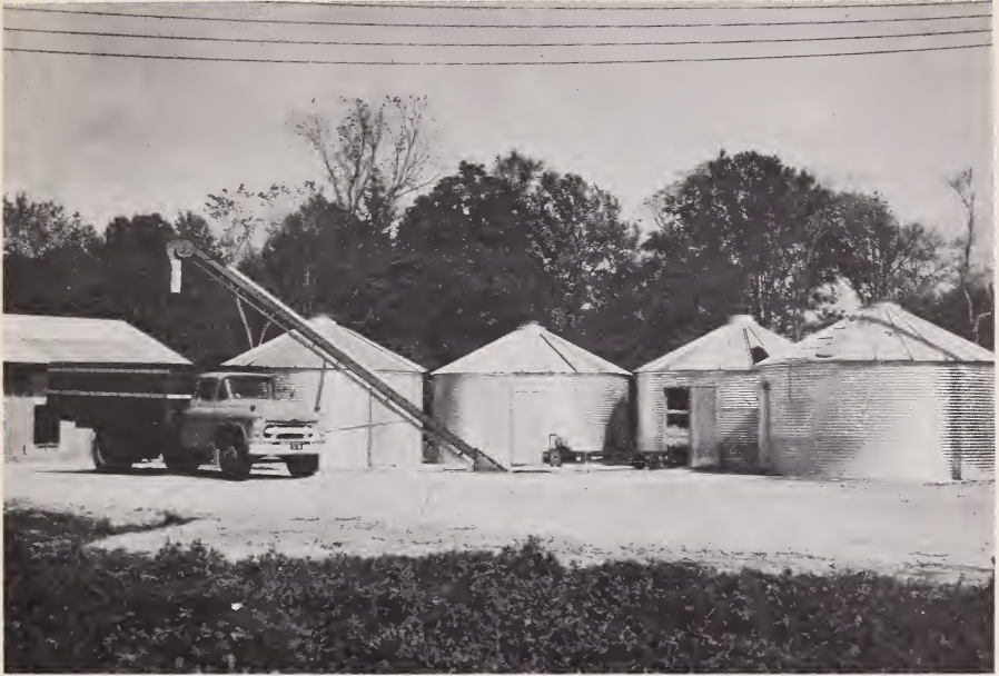
FIGURE 4.—Storage bins equipped with driers. Each pair of bins is serviced by one circulating fan heater (not in view). The heated air is blown up through the farmers' stock peanuts. The conveyer in front of the bins is on a turntable so it can be moved for loading and unloading any one of the bins.
