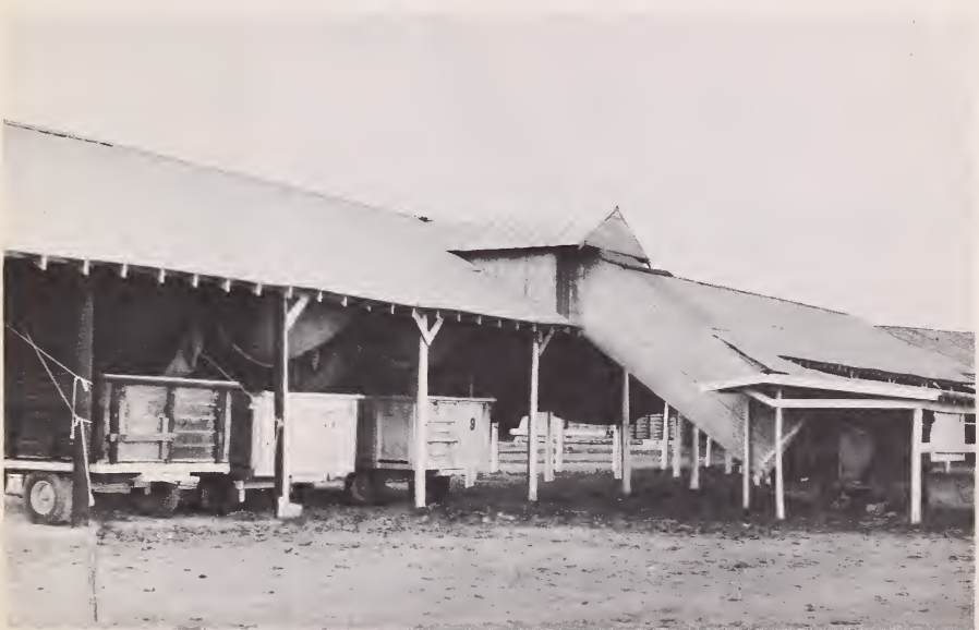
FIGURE 5.—Wagon driers with heating equipment for drying farmers' stock peanuts. Each of these wagons holds approximately four and one-half tons. A canvas hood fastens over the top of each wagon and air under controlled temperature is blown down through the peanuts. The bottom of the wagon is covered with heavy mesh screening to permit the forced air to escape.
