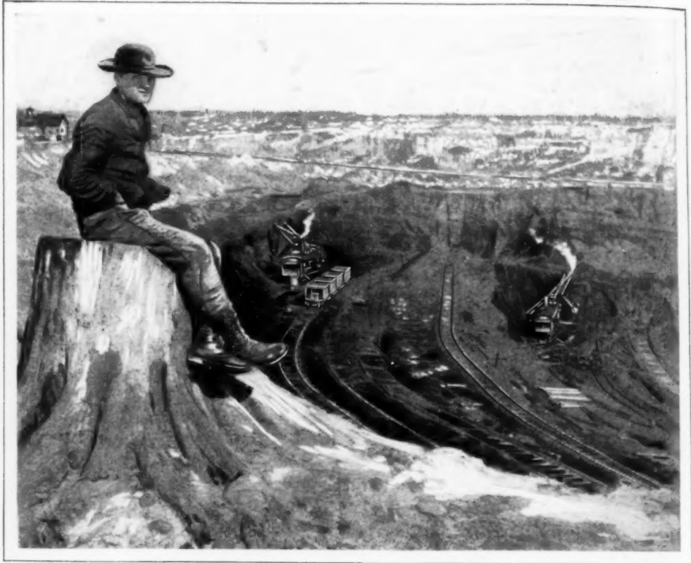
Part of the Burt Open-Pit Mine. One of the Big Ore Producers of the Mesaba Iron Range, in Minnesota; This Mine Has an Output of 10,000 Tons of Iron Ore Daily
