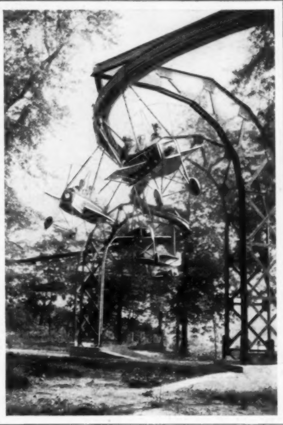
Airplane-Coaster Ride That Gives Many of the Thrills of Real Flying; Cars Are Propelled by Electricity
