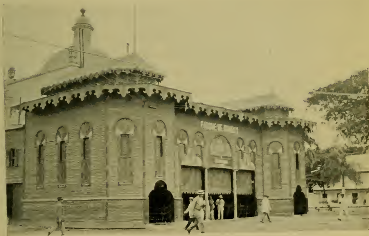
NEW DOCK, PONCE FIRE DEPARTMENT BUILDING, PONCE
