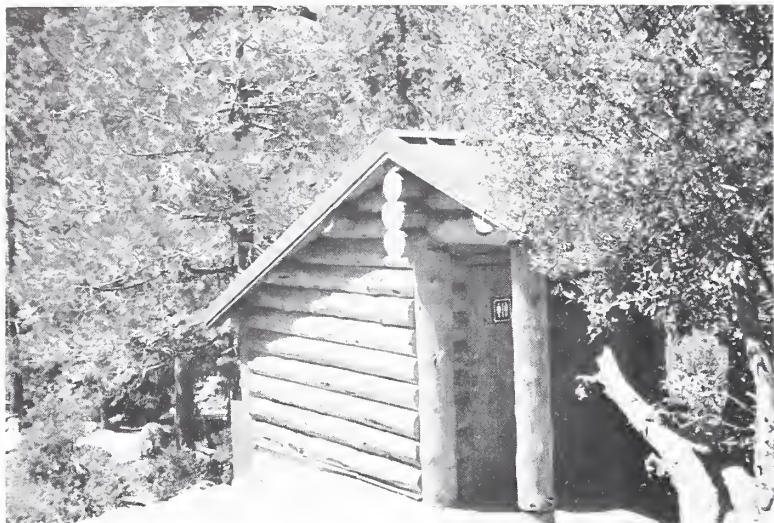
Figure 13. Yosemite site fabricated compost toilet at Nevada Falls, front view.
