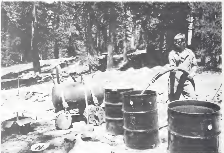
Figure 27. Pumping a septic tank. The sludge is pumped into barrels, then flown out of the backcountry.
