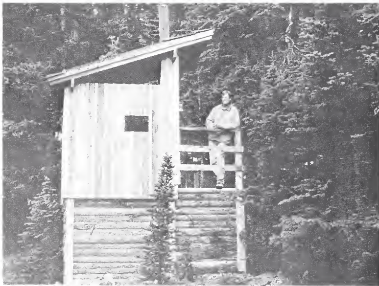
Figure 15. Sunergy Systems LTD. building at Yoho NP (Canada) for a Phoenix digester, side view.
