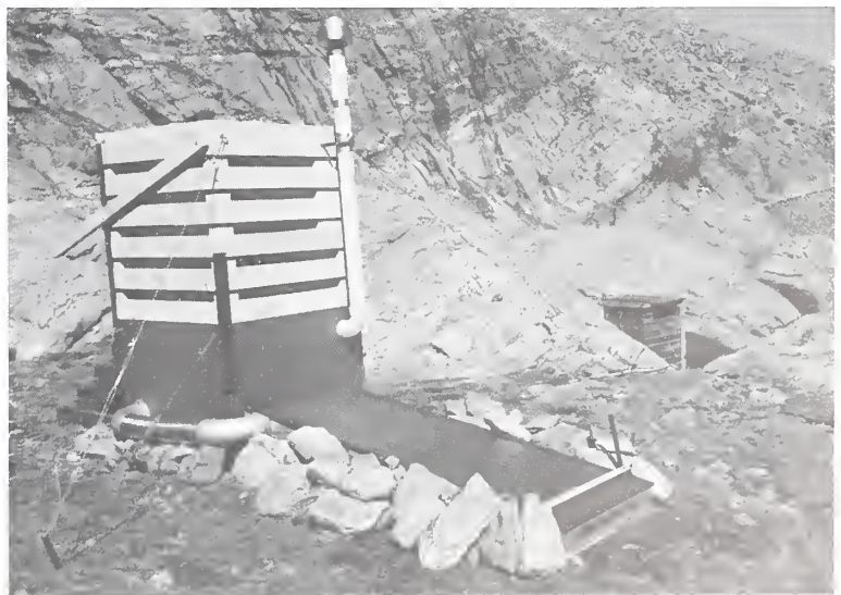
Figure 24. Rocky Mountain dehydrating toilet, back view. The heat collector is located below basement. Liquid evaporator is behind the hill.
