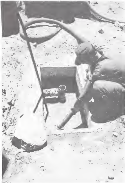
Figure 25. Pumping a septic tank in the backcountry.
