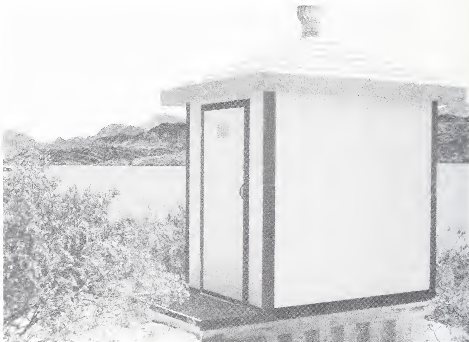
Figure 20. Trail-head toilet. The building is by Restroom Solutions, Inc. (RSI), with a Clivus Multrum direct burial compost digester.
