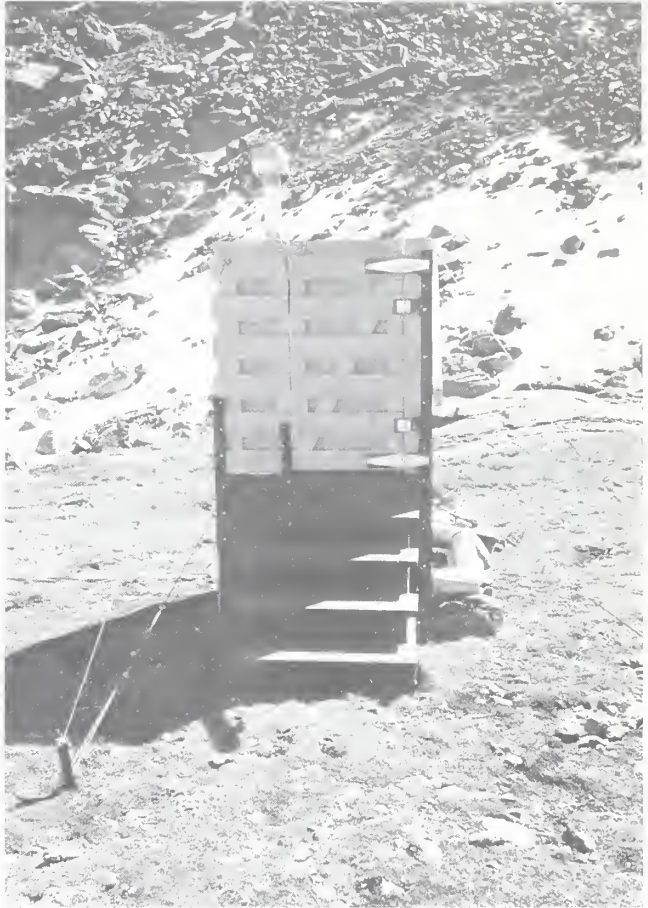
Figure 23. Rocky Mountain dehydrating toilet at Chasm Meadows, front view. Elevation 11,500 feet. Guy wires are needed due to high winds. Four-sided privacy screen is used to keep building height to a minimum.
