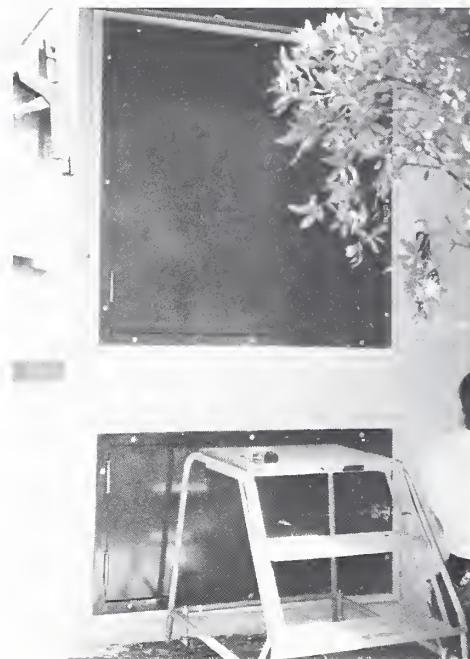
Figure 14. Yosemite compost toilet, basement view. Double doors to basement open to allow easy access to the maintenance and clean-out areas of the digester.
