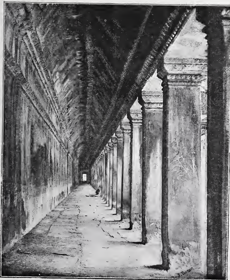
SECTION OF AN OUTER GALLERY AT NAKHON WAT.
