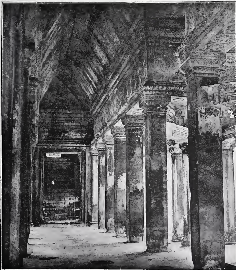
ELEVATED COLONNADE LEADING TO CENTRAL TOWER AT NAKHON WAT.
