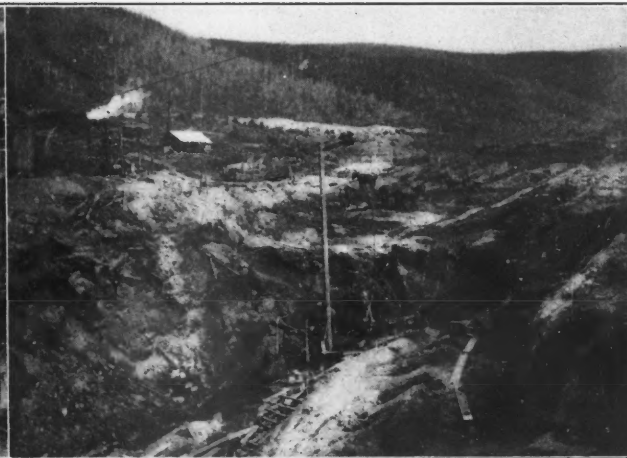
FIG. 10. HORSE SCRAPING AND OPEN CUTTING.
