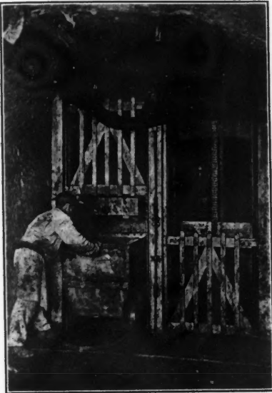
STATION LANDING IN COURRIERES MINE.
