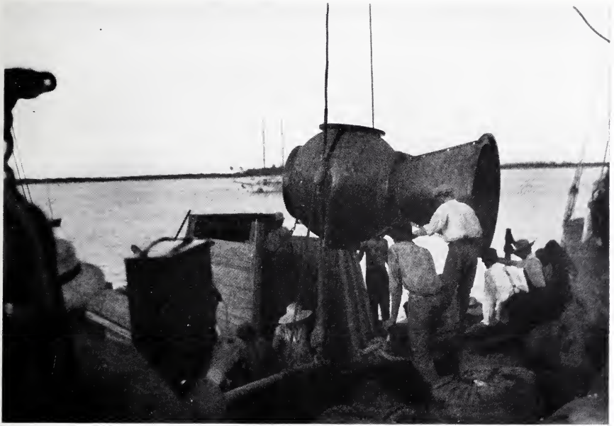
PHOTOGRAPHER'S CHAMBER BEING PLACED ABOARD BARGE
