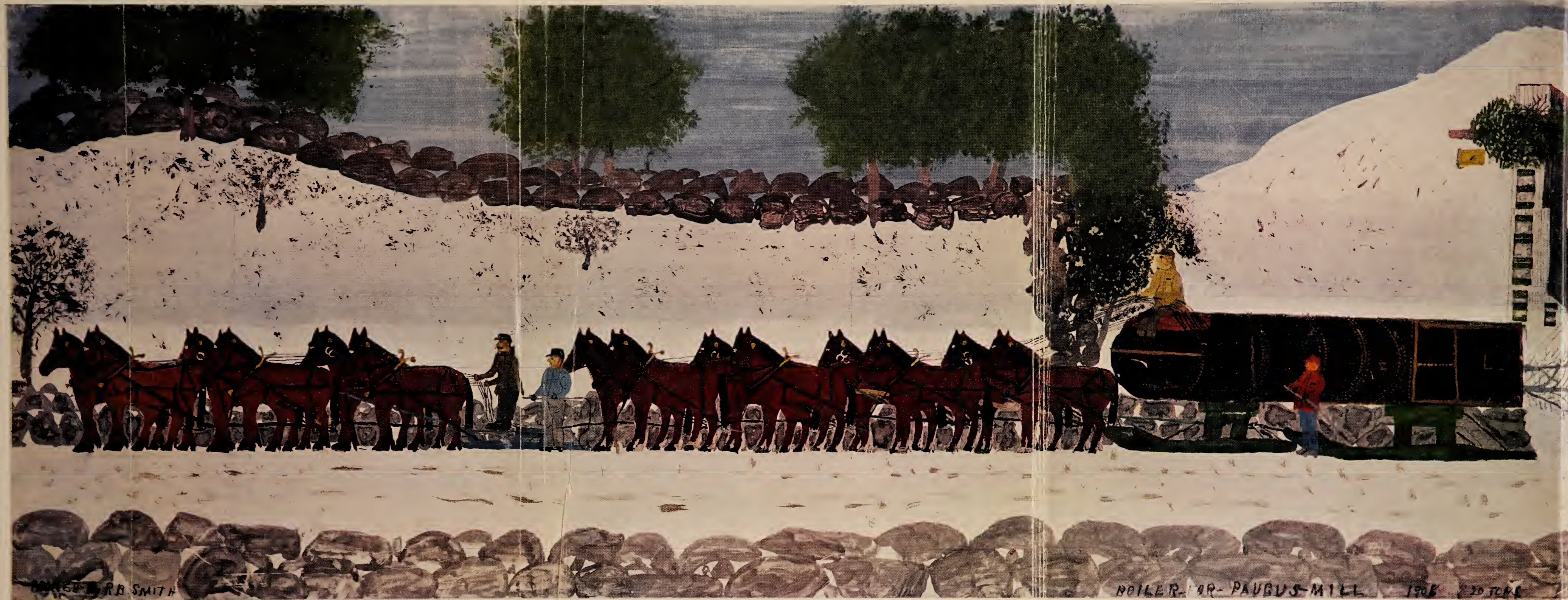
BOILER BEING TRANSPORTED FROM FREIGHT DEPOT UP TO PAUGUS MILLS
