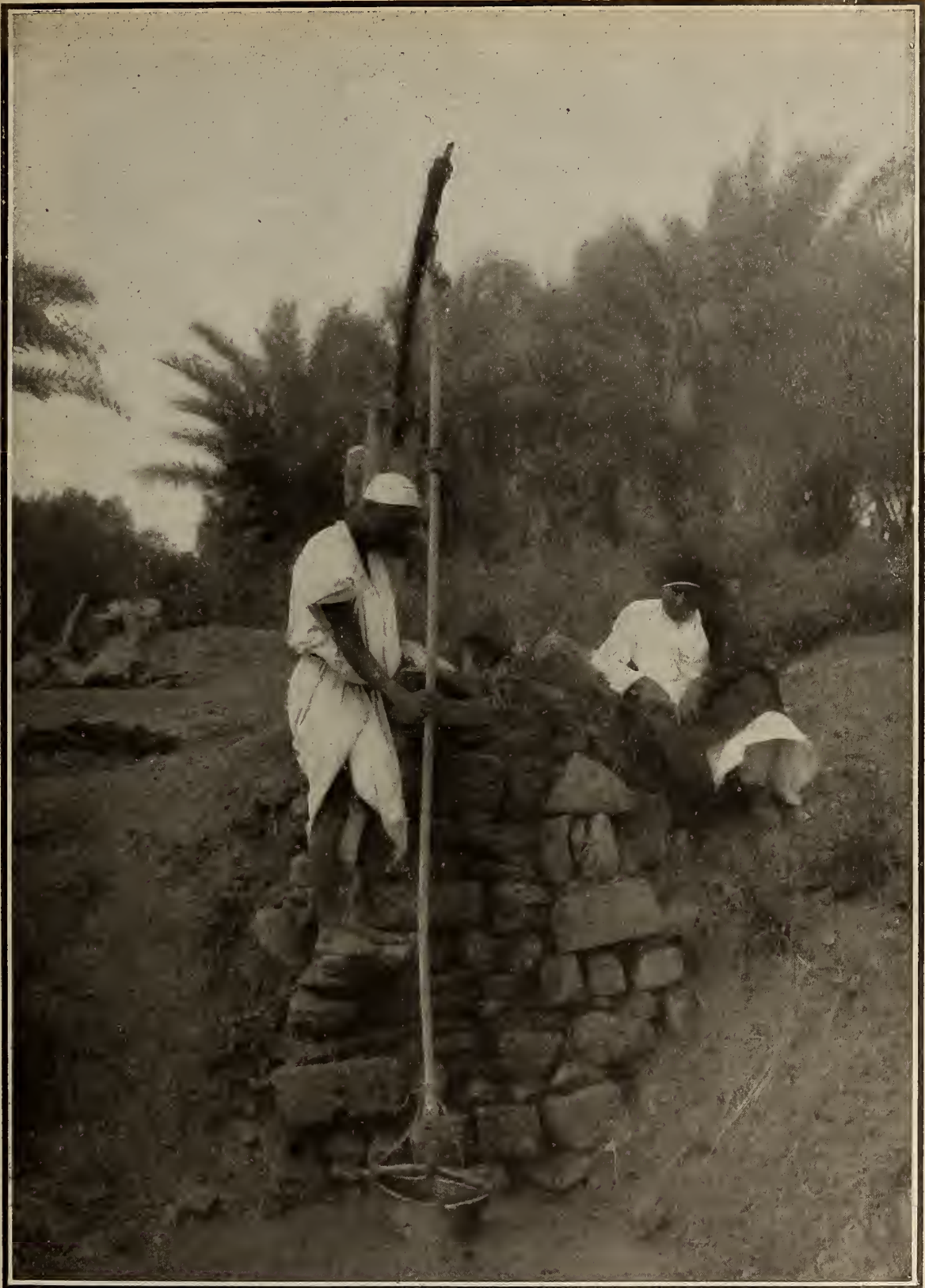
OLD WAY OF GETTING WATER OUT OF THE NILE. (Gen. 41:1.) We see in the above picture the slow and tedious way the Egyptians have of getting water out of the river Nile. The process is by hand with the aid of a sweep pole. This is very different compared with the modern way of throwing the water up over a wheel, which is turned by oxen. We notice that improvements have been very slow among the people in the land of the great pyramids; however, the Egyptians were more interested in building tombs and pyramids, than in making progress in other lines, which would have lessened labor and added much more to the comfort of the people.
