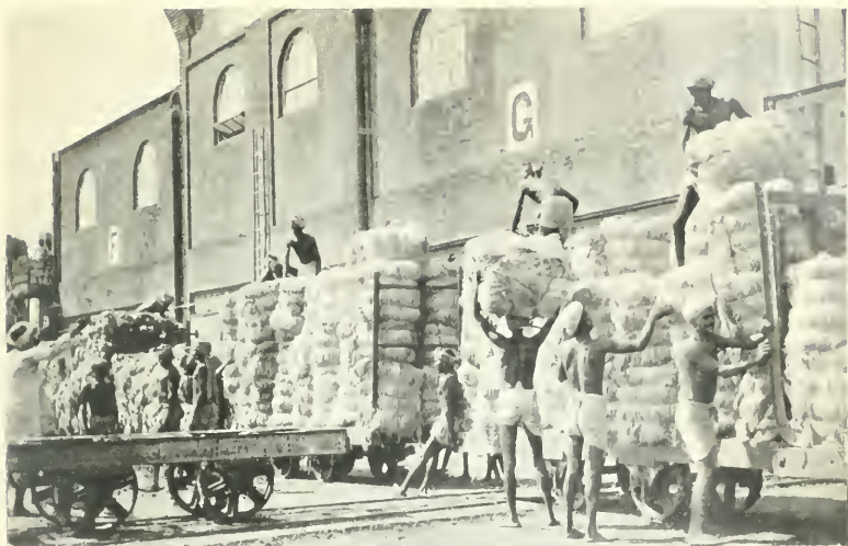
LANDING JUTE AT NARAINGUNJ.
