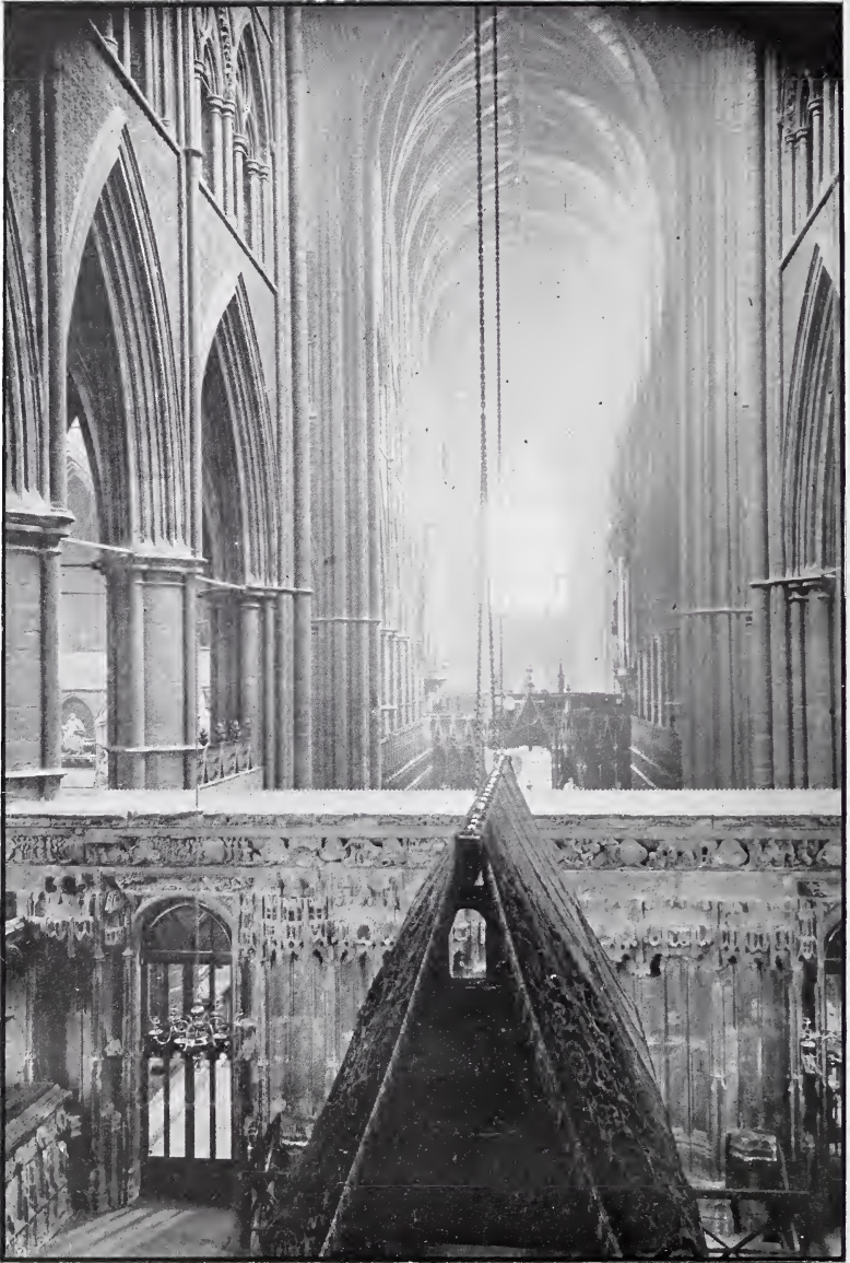
Interior from East
