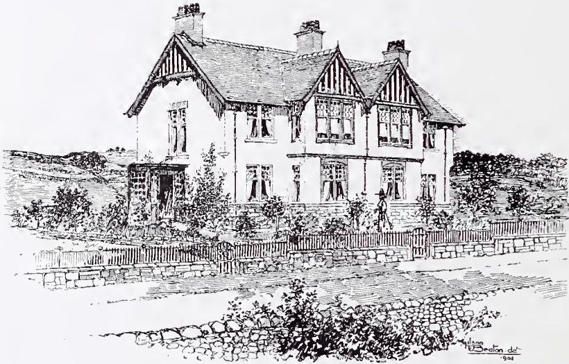
574. Residences at Kilmalcolm, JAMES AUSTEN LAIRD, Architect.
