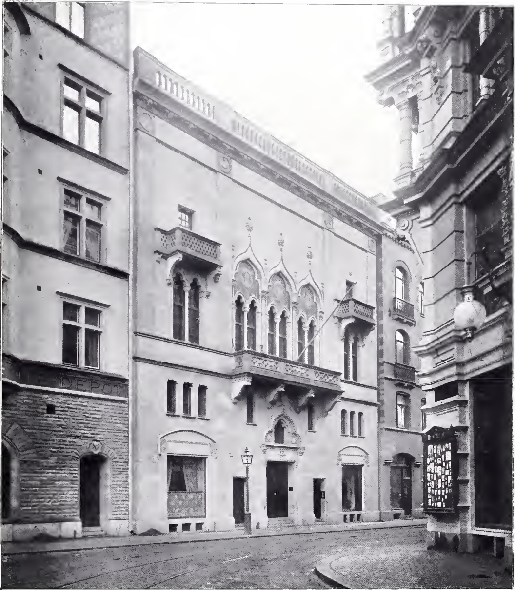
House of the Swedish Artists' Association, Stockholm, LUDV. PETERSON, Architect. (For Plans, see p. 136.)
