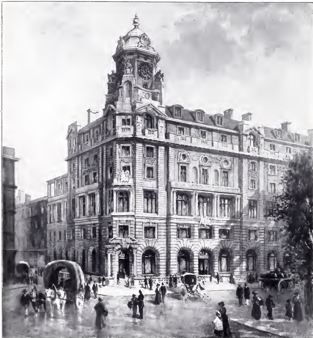
1452. Royal London Friendly Society's New Building, Finsbury Square, E.C., JOHN BELCHER, A.R.A., Architect.
