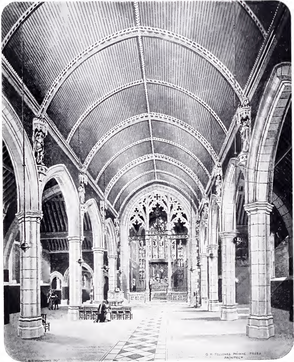
1583. New Church, Belvedere, Kent, Interior View, looking East , G. H. FELLOWES PRYNNE, Architect.
