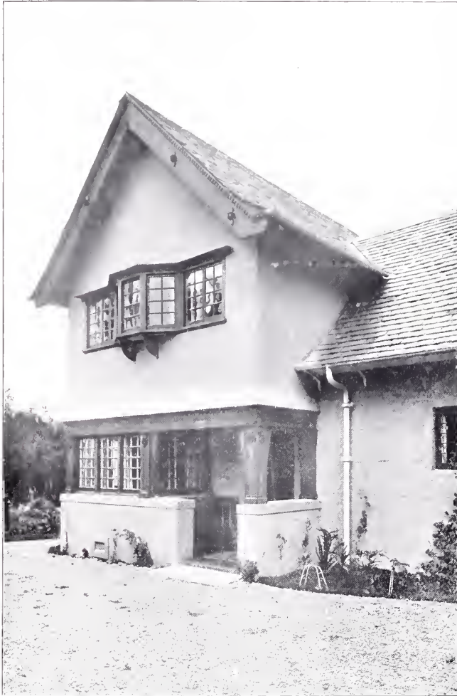
548. Gable of Duneryne Cottage , JOHN A. CAMPBELL, Architect.
