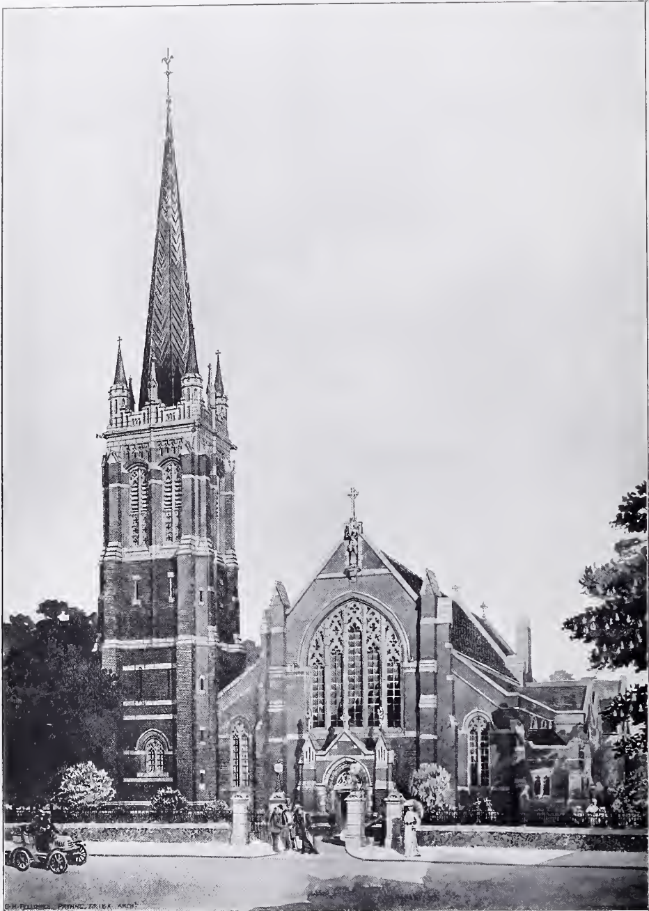
New Church, Belvedere, Kent, Exterior looking West, G. H. FELLOWES PRYNNE, Architect.
