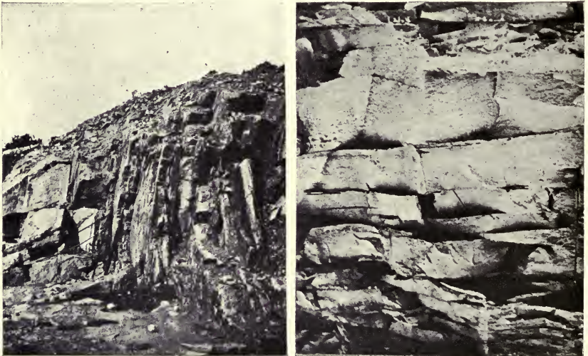
FIG. 48.—Vertical and horizontal joints in granite, Conn. (U. S. Geological Survey.)
