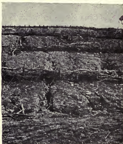
FIG. 116.—Checking of soil erosion by brush dams. (U. S. Geological Survey.)
