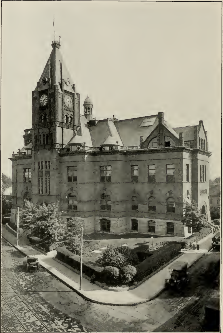
BROCKTON CITY HALL Dedicated, 1894
