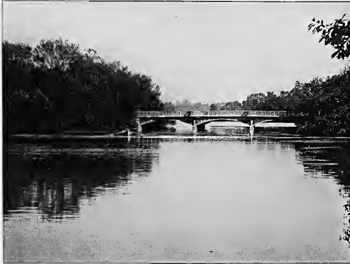
BUFFALO PARK BRIDGE.
