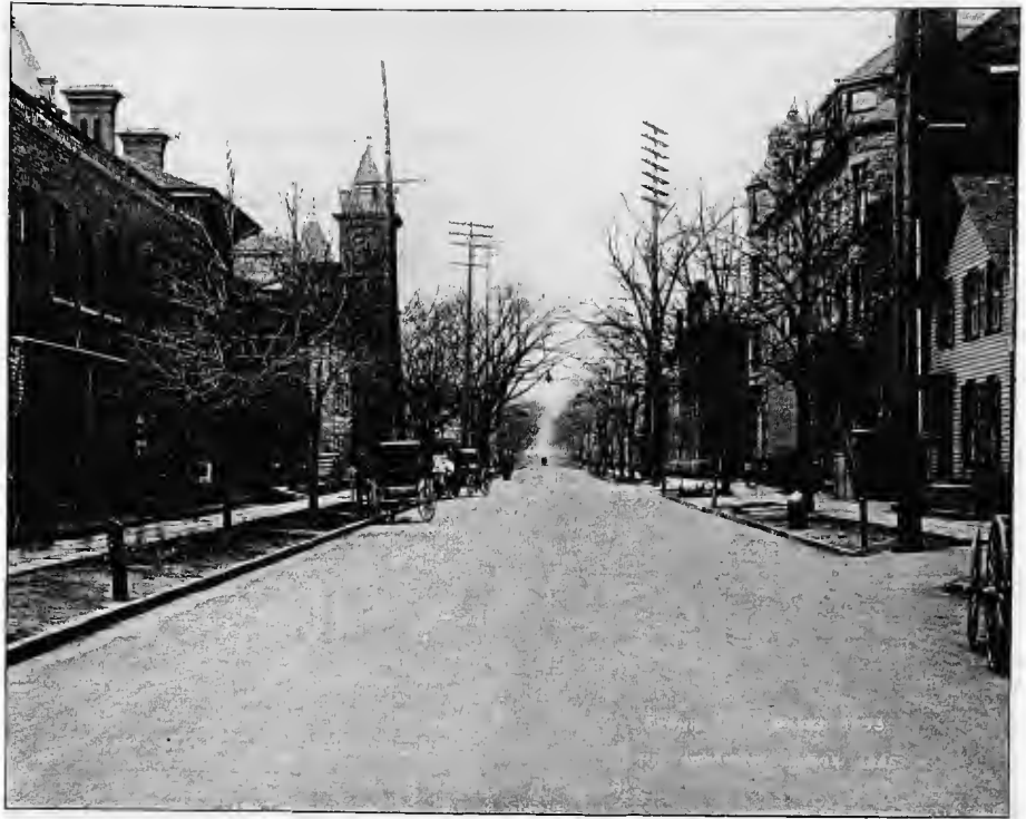
FRANKLIN STREET, LAID WITH TRINIDAD ASPHALT PAVEMENT.
