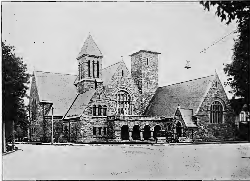
THE NEW FIRST PRESBYTERIAN CHURCH.
