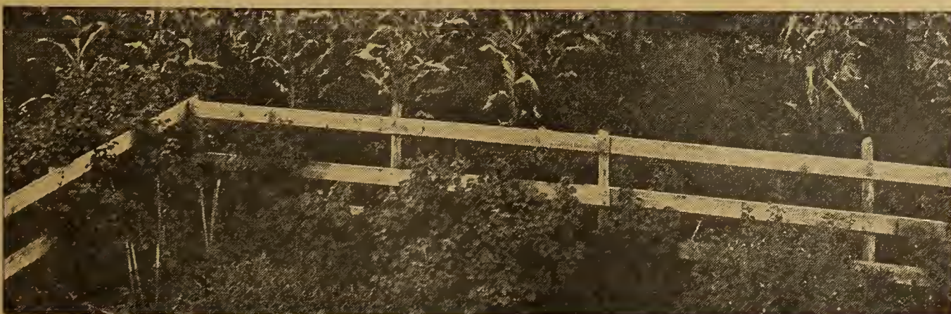
Don't let weeds grow around your fences like this. They make the posts decay
