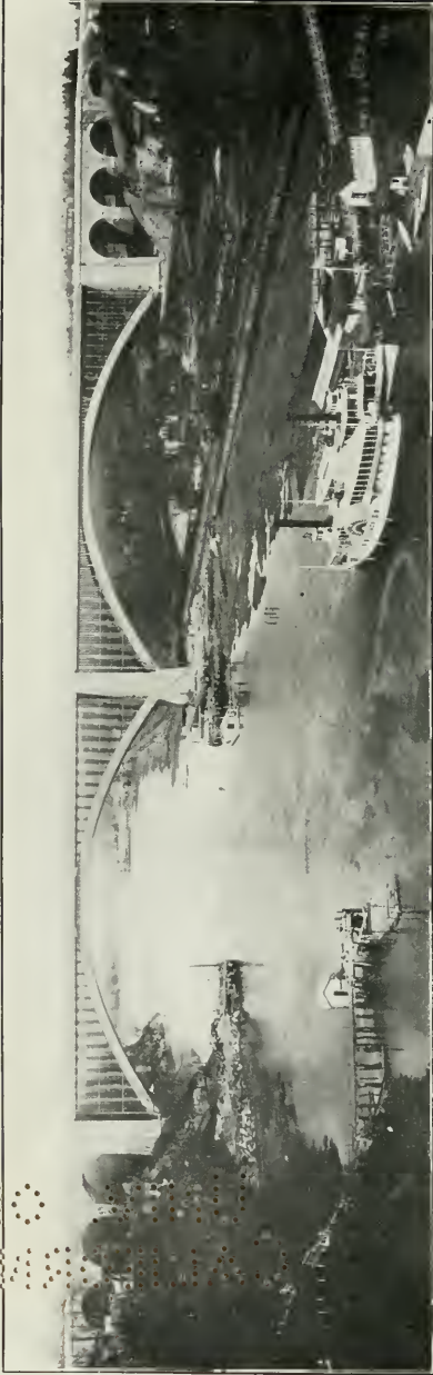
WASHINGTON BRIDGE, HARLEM RIVER, NEW YORK. Steel Arches, 510-ft. Span ; Stone Arches, 60 ft. Span.
