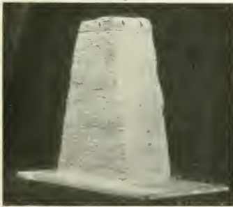
FIG. 163. Tower of Oxford Castle.
