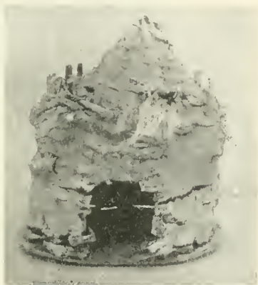
FIG. 72. British Hut daubed with Clay.
