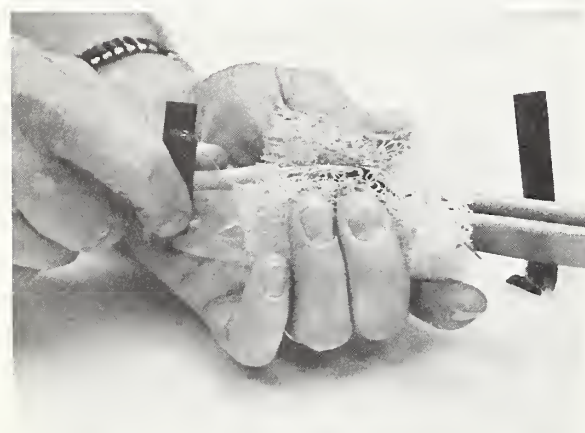
B.— Position mold around splice.
