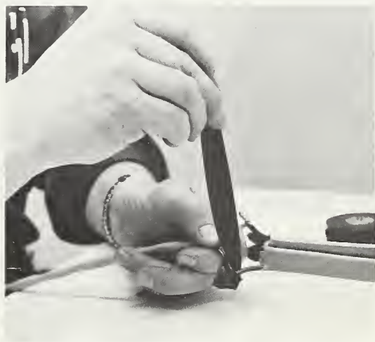
E.— Wrap with rubber splicing compound and plastic tape.
