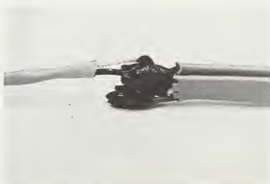
F.— Properly taped splice.
