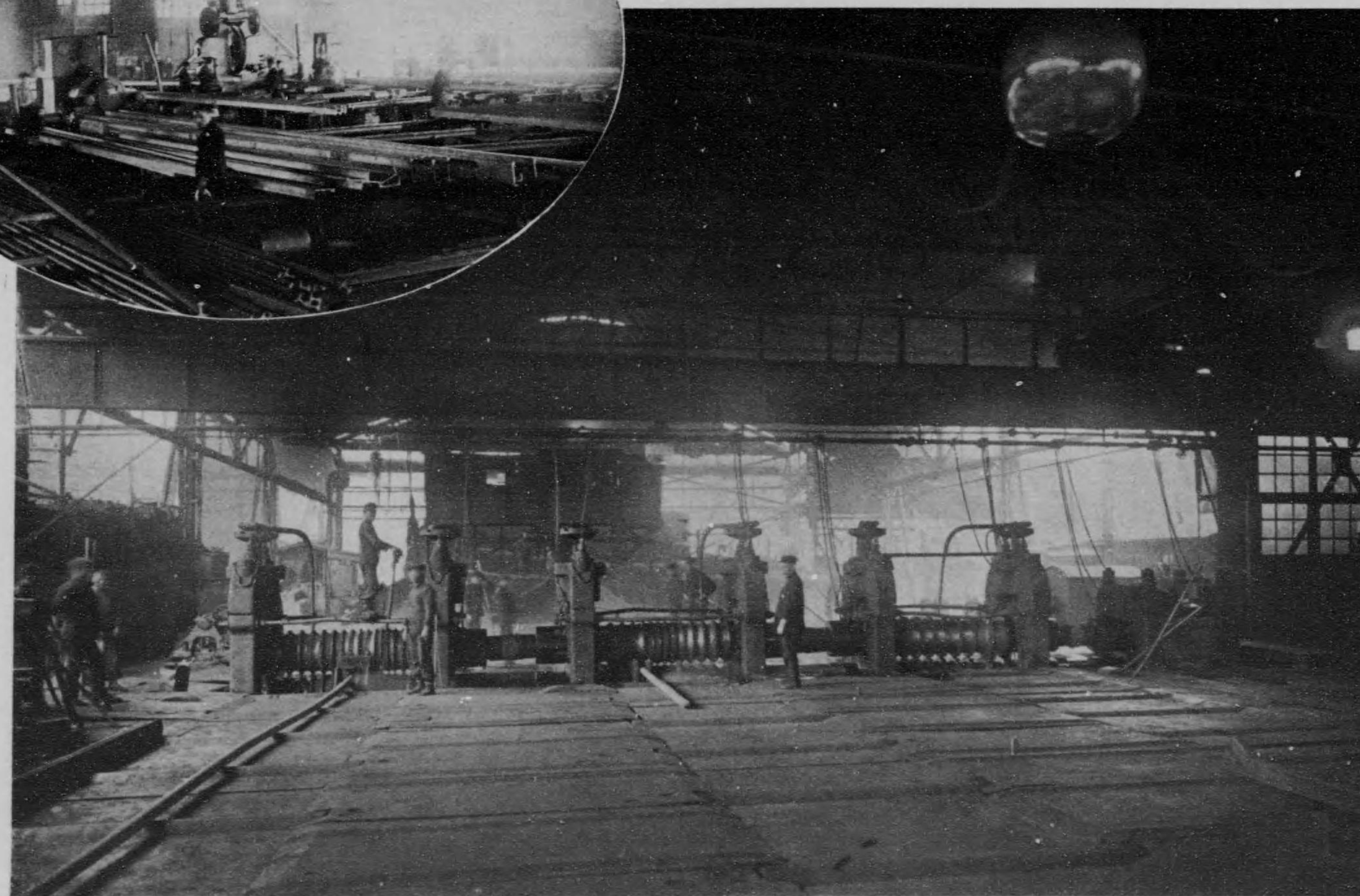
場工整精之機ル一口形大 LARGE BAR MILL AND FINISHING SHOP.
