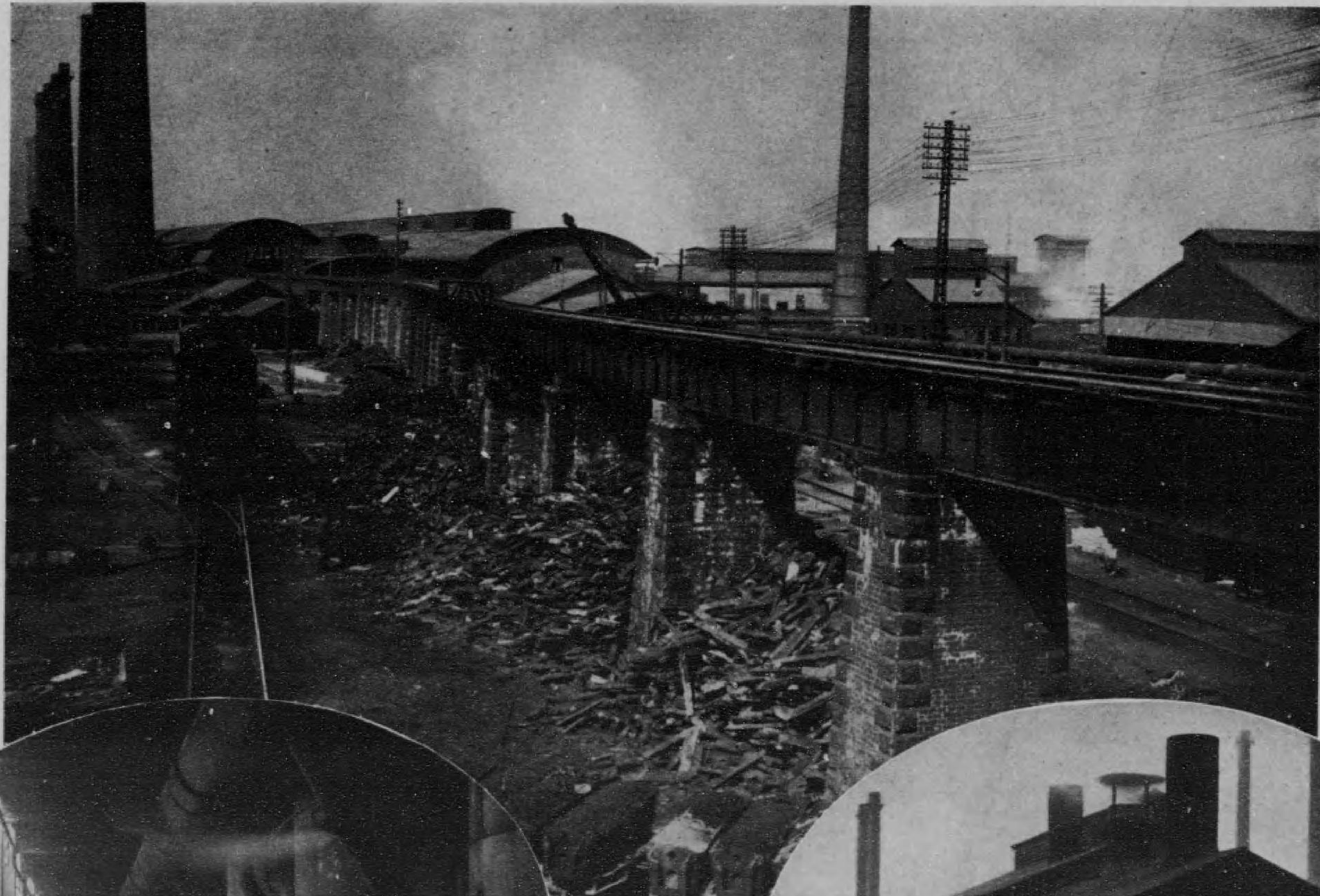
場置鐵屑 SCRAP YARD.
