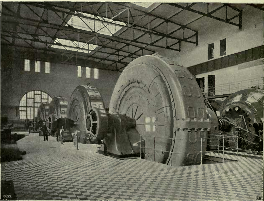
INTERIOR OF WATER- POWER STATION AT TROLLHÄTTAN
