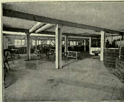
INSPECTION ROOM FOR TUBES.
