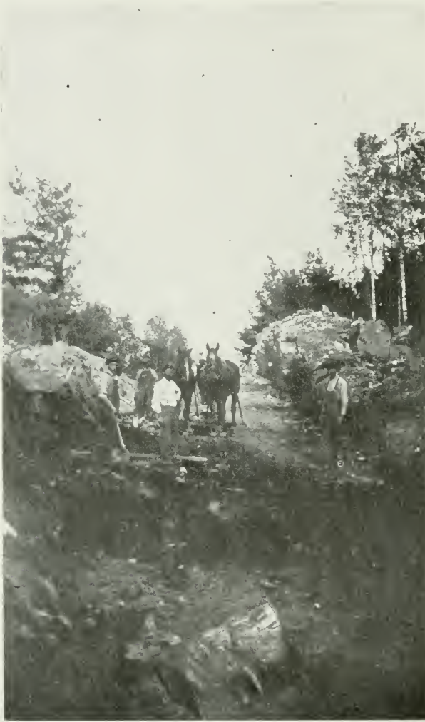
Road Construction in Muskoka.
