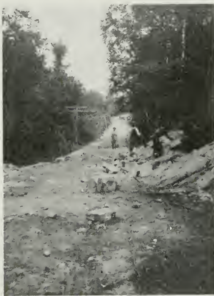
Severn to North Bay road widening.
