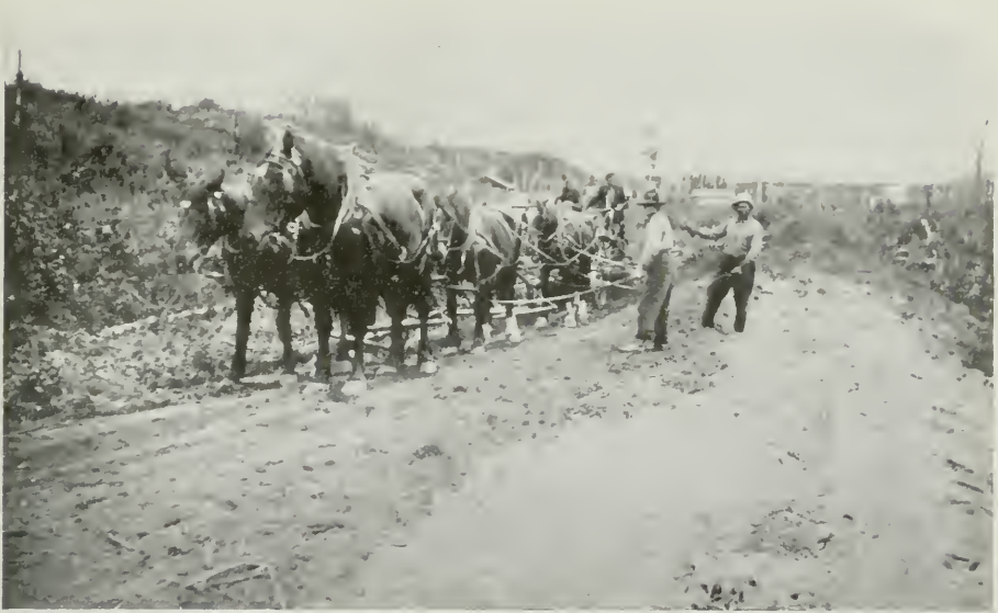
Grading new road, Northern Ontario.
