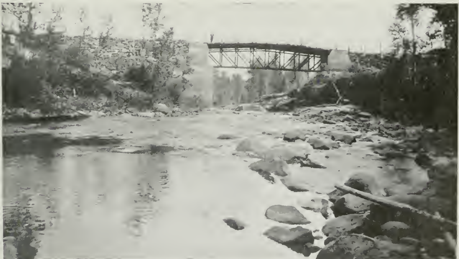
McKenzie River Bridge, Northern Ontario.
