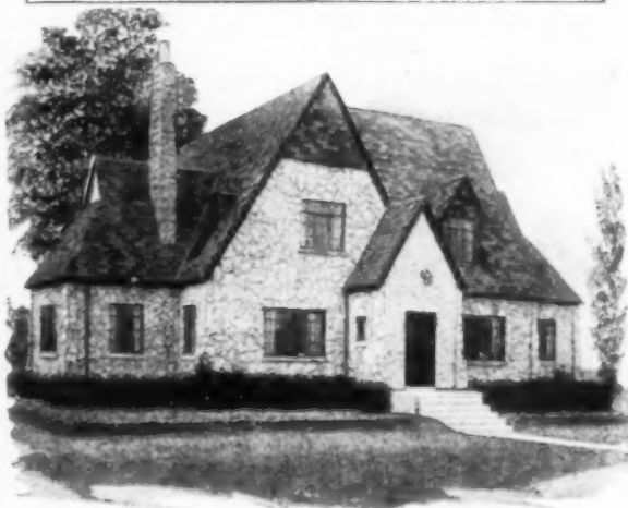
Top to Bottom. Finishing One of the Walls, Hoisting It, and View of Completed House
