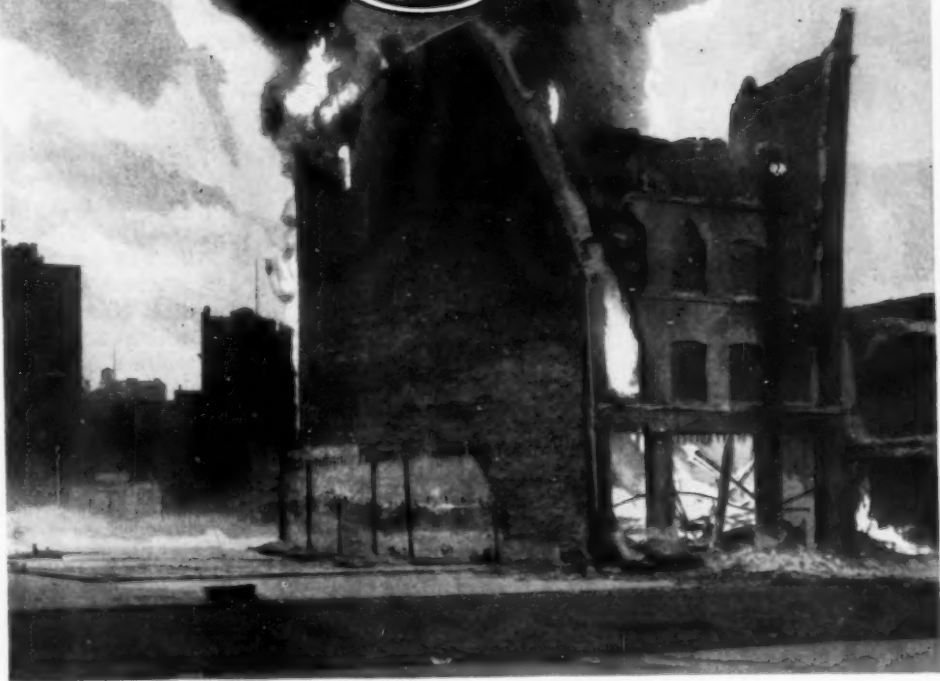
Just as the Walls Began to Fall; a View of the Five-Story, Washington, D. C., Building Burned by Government Scientists to Study the Effect of Fires on Office Safes
