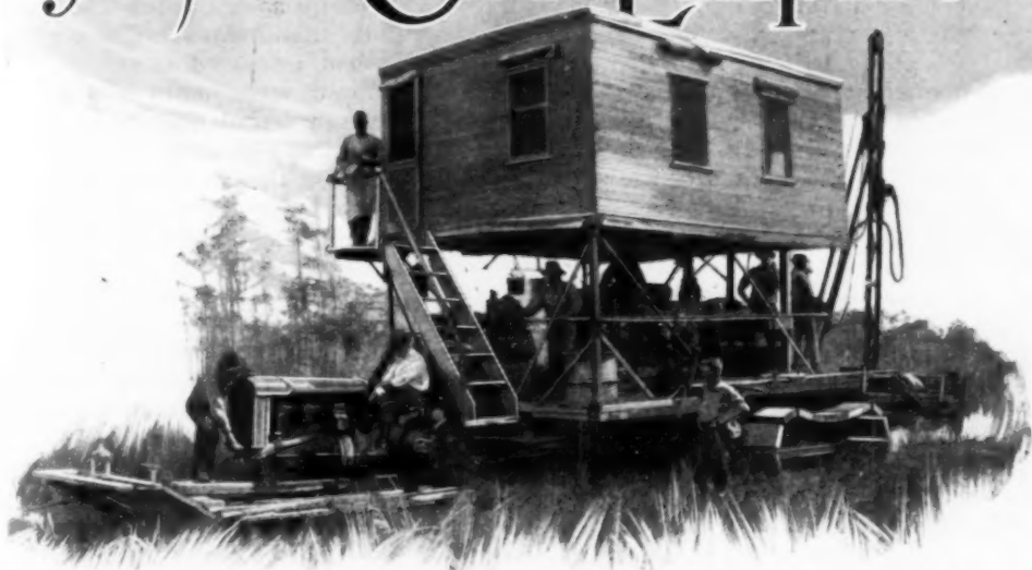
Combination Dynamite Drill, Stump Puller and Traveling Cook Shack, One of the Unique Tools Used to Build the Tamiami Highway through the Wilderness of the Everglades Jungle
