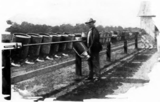
Rack Constructed from Lengths of Pipe Facilitates the Draining and Airing of Milk Cans
