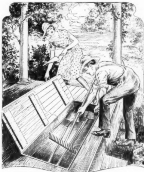
Handy Cabinet for the Garden Tools Can Be Built in the Porch Floor
