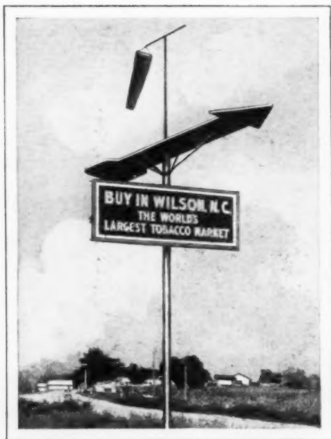
For the Guidance of Airmen, This Sign Shows the Wind Direction and Points to Town
