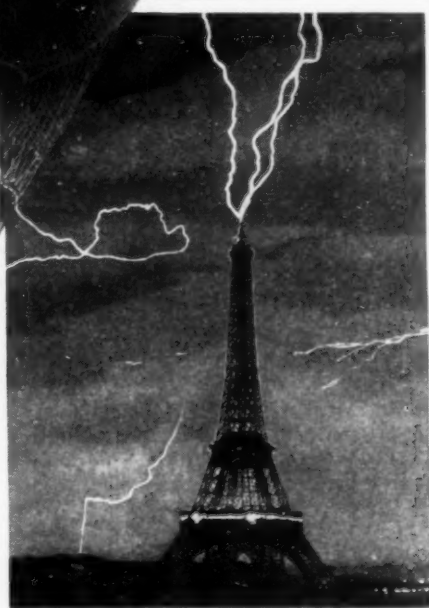
The World's Tallest Lightning Rod, the Thousand-Foot-High Eiffel Tower in Paris, Photographed Just as It Was Struck in a Storm
