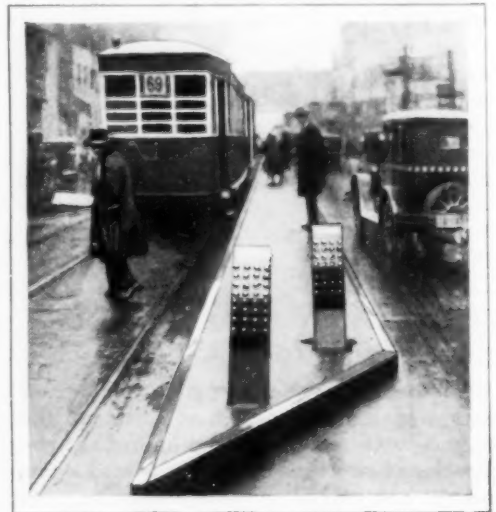
"Cat's Eye" Lights on Safety Guards at Street-Car Loading Station Help Protect Passengers
