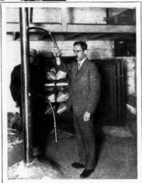
Rigging the Thermocouples, Setting an Alarm Clock in One of the Safes, and, Bottom, the Basement-Debris-Temperature Takers
