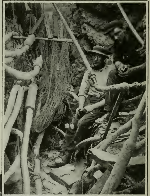
The only cable cut. It was necessary to do this to get around an obstruction. There were 800 wires to be cut and spliced individually
