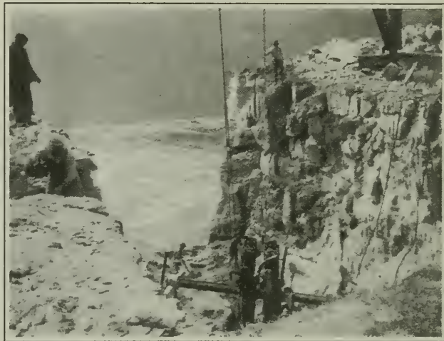
Heavy rock excavation at Thompson's Point. The Whirlpool appears below
