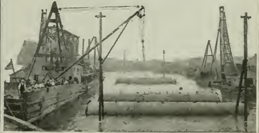
A section ready to be launched for towing to its resting place. Note the great size by comparison with the man
