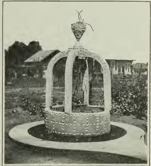
Shells make concrete decorative in detail as well as in line
