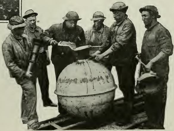
Loading an American mine. Unanchored automatic or floating mines must be dead in an hour. Various devices are incorporated to obtain this result
