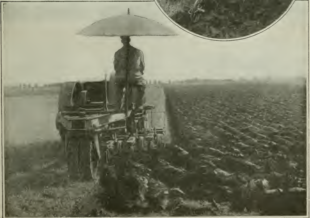
Below, a self-contained motor plow of the latest type, cutting three furrows at once. This illustrates one of the great advantages of the tractor, for it can really do multiple work, day after day, and with absolute reliability. Nothing but the worst sort of weather can stop it or delay its work
