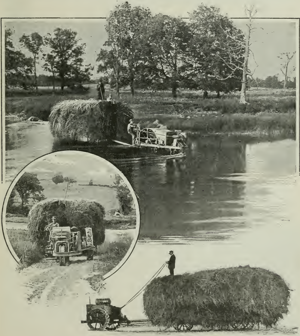
A real gasoline horse guided by reins. It can go anywhere and never gets tired
