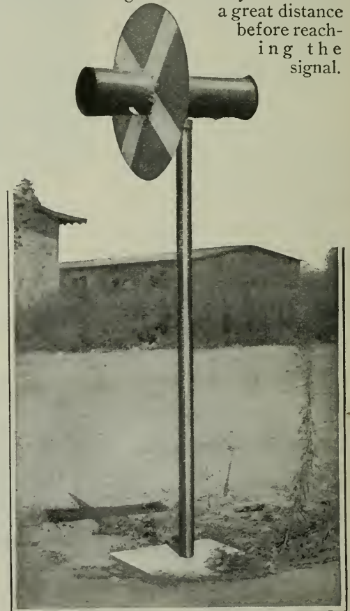
A red light inside the tube of this railway signal is visible for a great distance, and the disk attracts attention in the daytime
