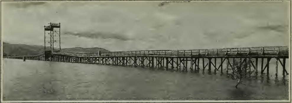
A bridge, two miles in length and twenty feet wide, is stretched across Pen d'Oreille Lake, for the use of farmers who sell their produce in Sandport, Idaho
