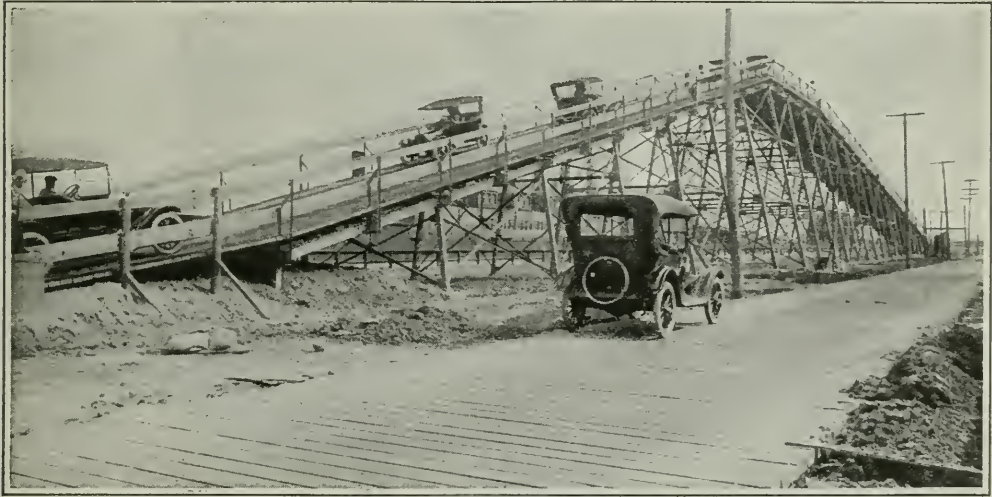
Detroit automobile dealers had to build this steep hill to order so as to have grades where they could demonstrate the hill-climbing proclivities of their cars in that city of level highways
