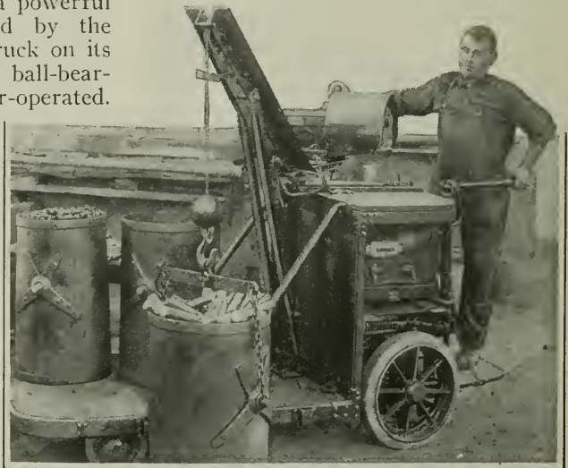
This truck runs around the shop and picks up and transports barrels and castings
