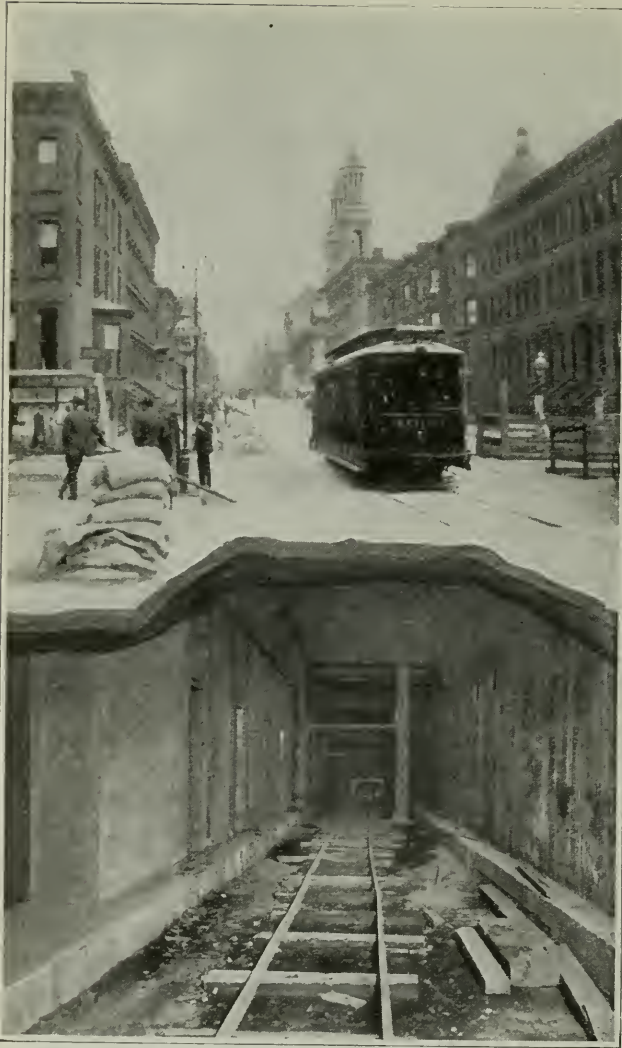
The new local tracks beneath Lexington Avenue near 74th Street. It will be noticed how free the street is from serious obstruction. This system, extended in a single track, would reach from New York's city hall into the borders of Eastern Tennessee, some six hundred and twenty-one miles
