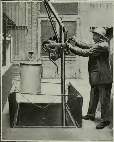
Rubbish removal is slowly being modernized. Here is the newest form of collapsible derrick for city houses
