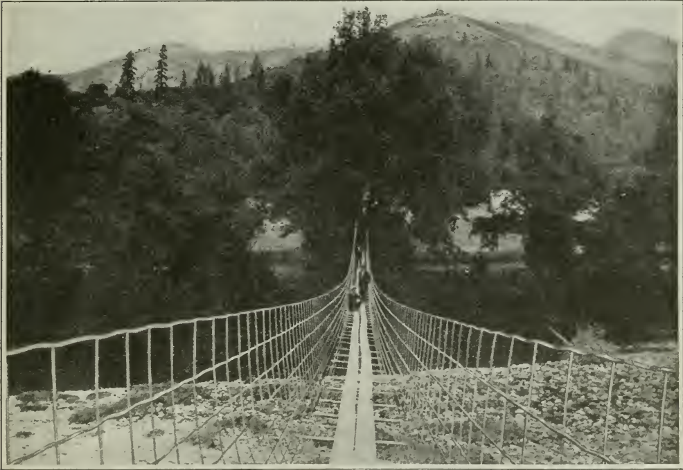
Suspension bridge built of fence wire
