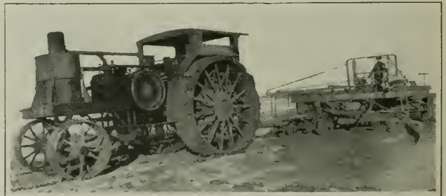
A traction engine pulls the machine which performs the three functions of scraping, cutting and rolling
