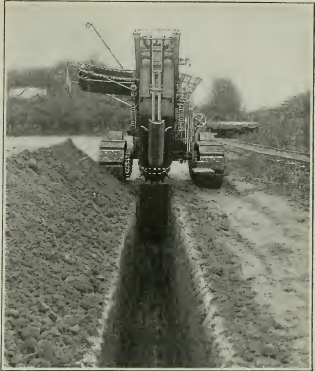
"Caterpillar" wheels enable the big machine to travel over soft ground
