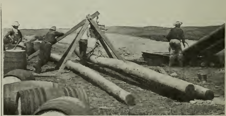
Before dipping in the preserving bath, telephone poles are weighed to determine whether or not they are well seasoned
