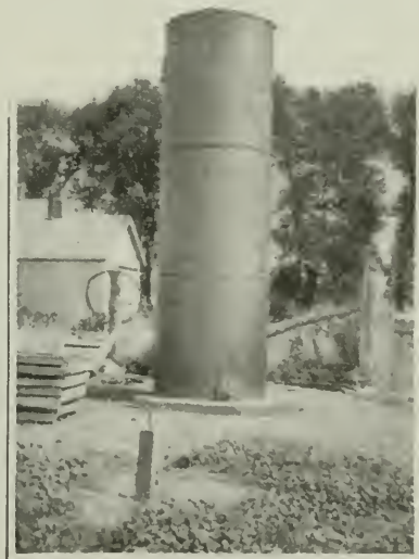
A farm stand-pipe made from an old boiler
