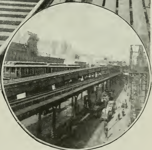
At each express station, the new tracks rise above the level used by the local trains
