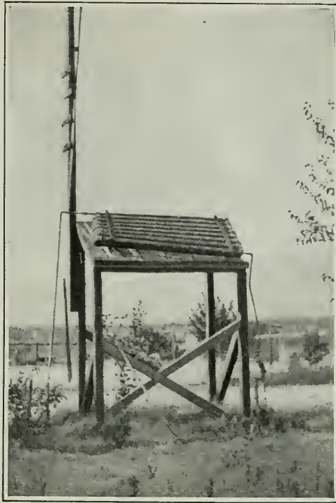
With this simple device the sun's rays are utilized to heat water
