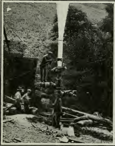
The gas blew off at a pressure of one hundred feet per square inch three feet above the outlet
