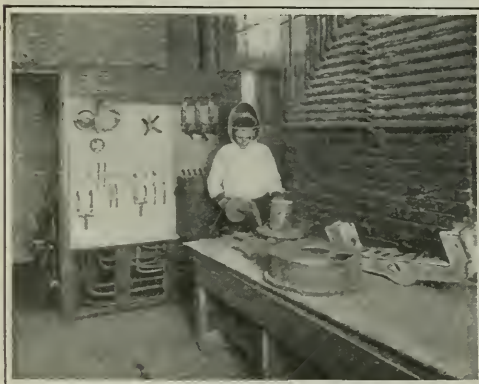
Broken or cracked castings can be quickly mended by means of an electric arc
