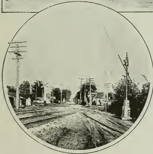
When the train approaches, a bell rings, a signal light flashes, and the arm of the pole drops down, thus lowering a number of heavy spiral wire tell-tales which should stop the most reckless motorist
