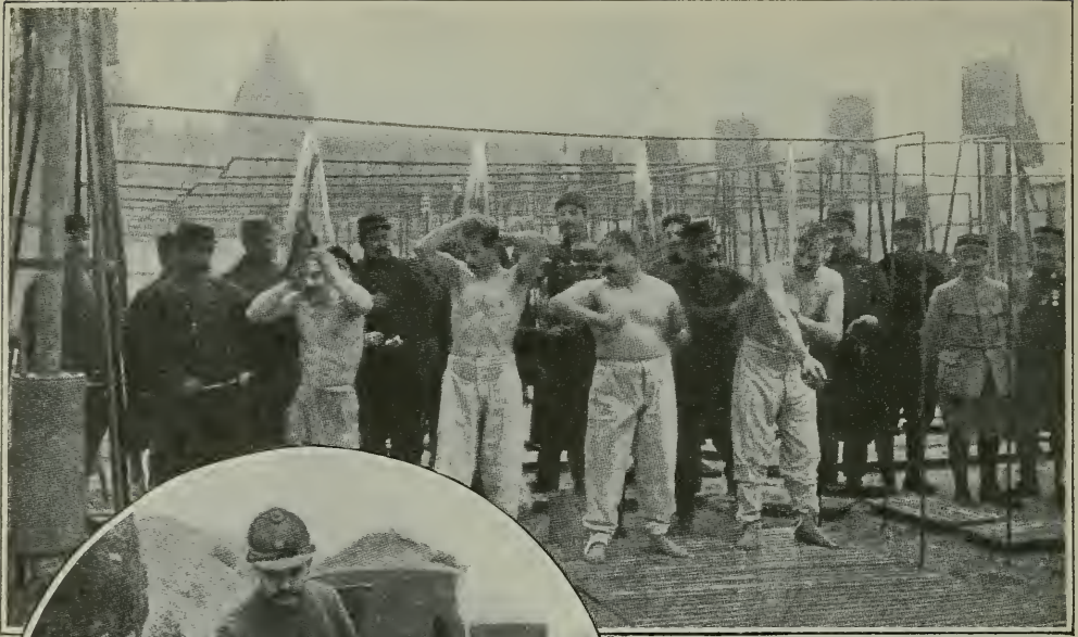
A large number of men can experience the luxury of a hot shower-bath by means of the arrangement shown above. The water passes through a heating apparatus before it reaches the spraying attachments
