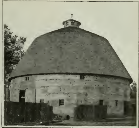
This round barn is made of reinforced concrete, eight inches thick. The loft has neither beams nor posts
