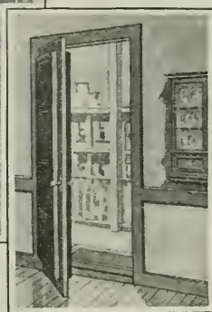
When the tradesman shuts the door of this receptacle, it can be opened only from the inside of the house
