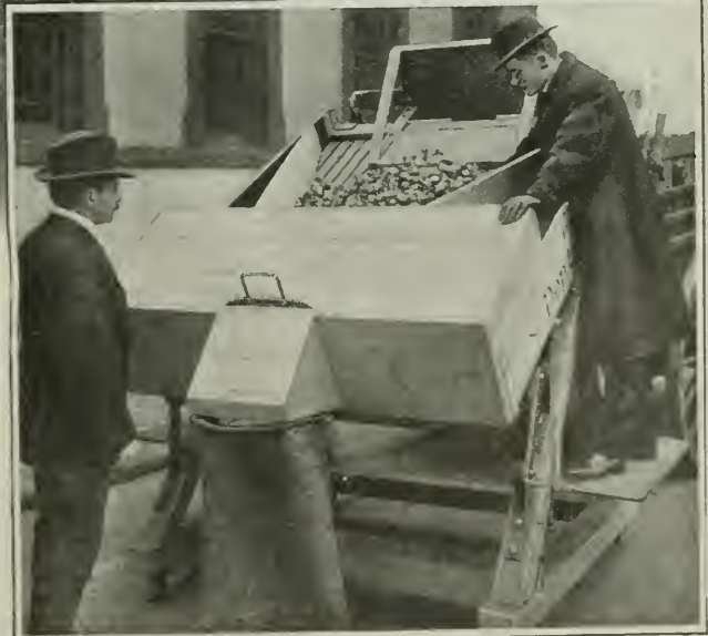
Each sack of vegetables or fruit can be dumped in the device, examined and re-sacked, all in a few seconds
