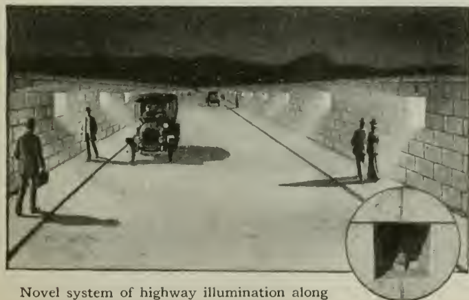
Novel system of highway illumination along the crest of the Kensico reservoir
