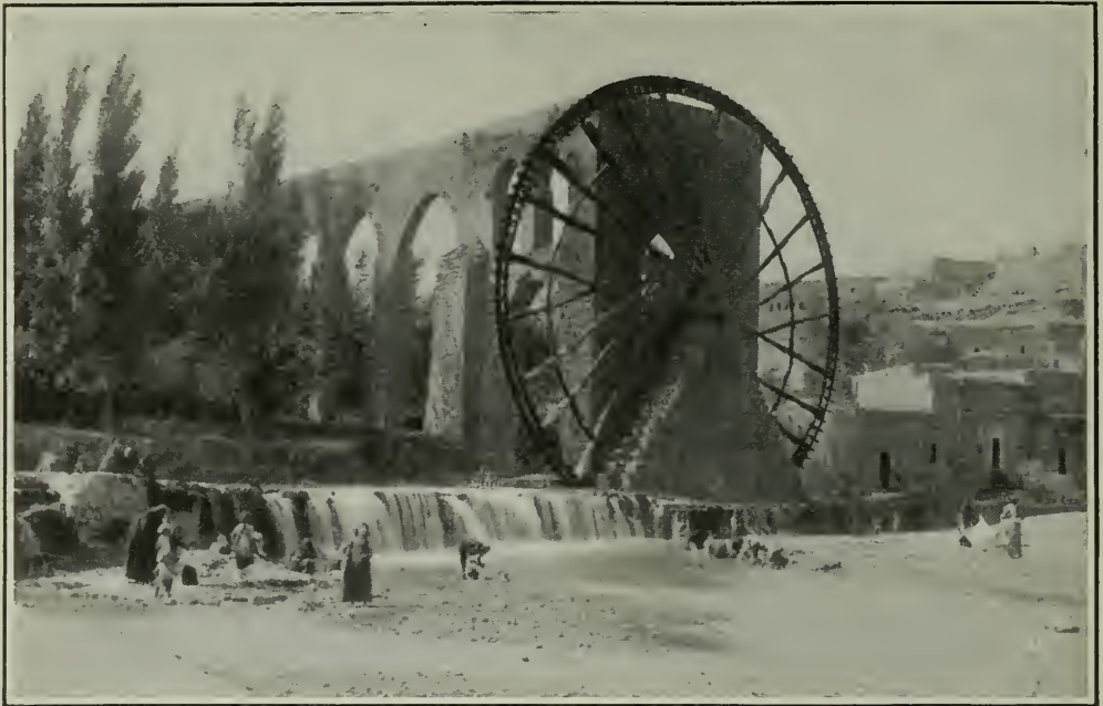
This ancient water wheel in Syria pumps the river up into the aqueduct at its top. Thus a wide territory is watered by other aqueducts and canals
