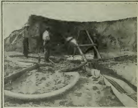
How the work was done. The hills were washed away with water which carried the mud formed down into the marshes
