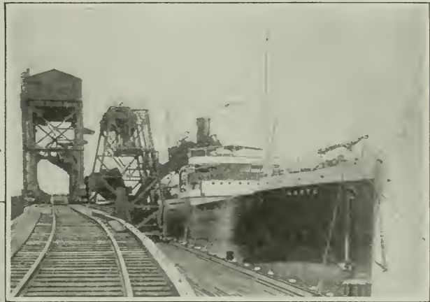
This giant coals steamers and loads barges by picking up railway cars and turning them upside down over the hopper
