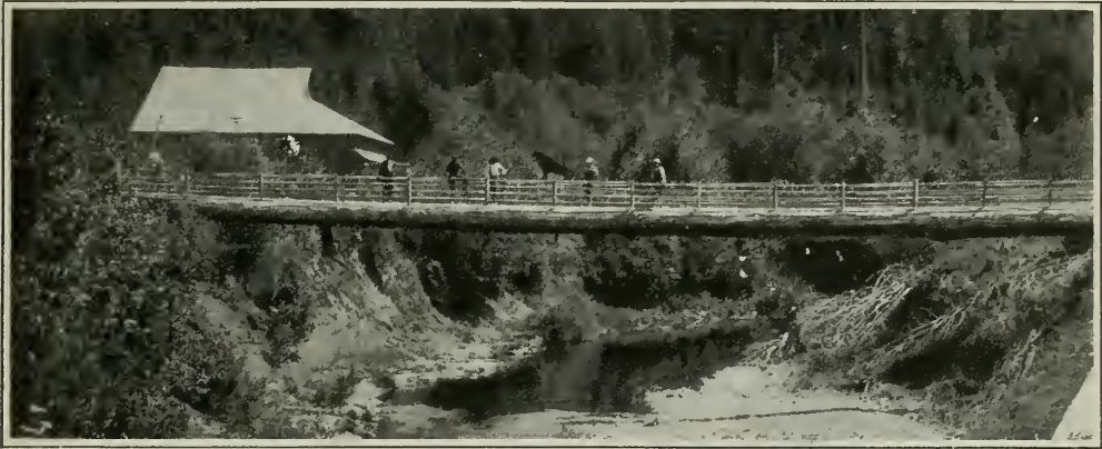
A giant fir, felled to drop across the stream, furnished this excellent foot-bridge
