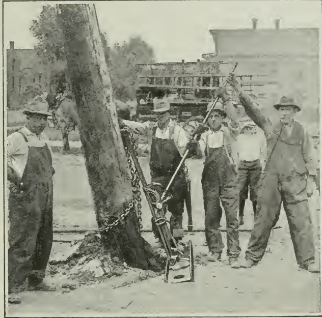
A pole was embedded five feet in the ground. It was removed by a powerful jack in four and one-half minutes exactly
