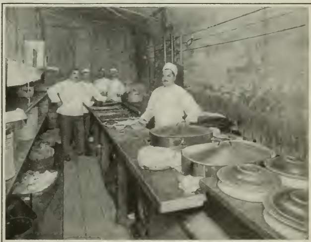
The underground kitchen in which the meal for a banquet given in St. Louis' new sewer was cooked
