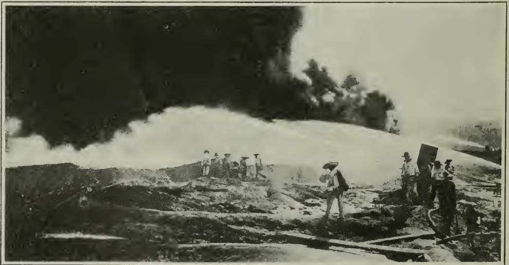
Pushing in the retaining wall which finally conquered the flames. The heat was so intense that streams of water had to be continually played over the workers, all of them Mexican peons, who are perhaps the most sensitive of human beings to extremes of heat and cold—except in their horn-like nether extremities, which were not affected in this case
