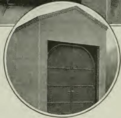
It formerly took weeks to paint and dry a railway car. With this oven it can be done in as many days
