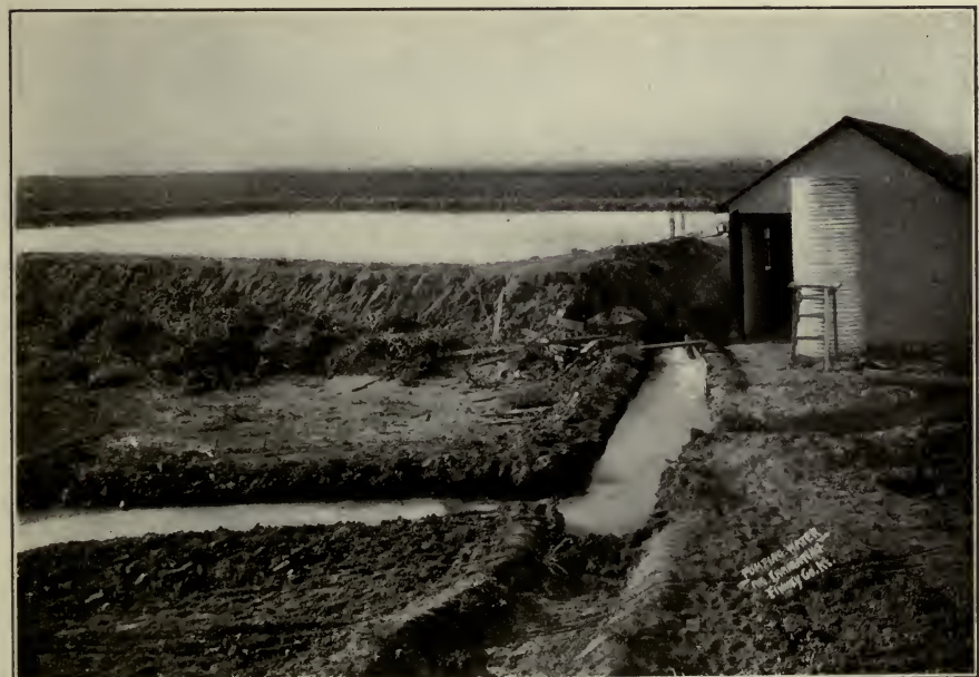
FIG. B.—Gasoline pumping equipment, delivering water into small earth reservoirs.
