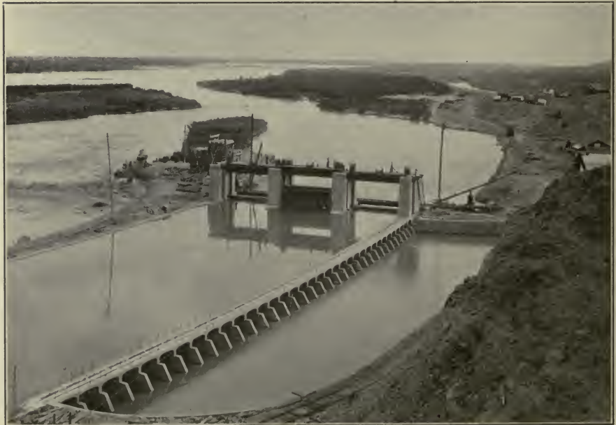
FIG. D.—Concrete headworks with sluice gates at Laguna dam on Colorado River, Ariz.-Cal.
