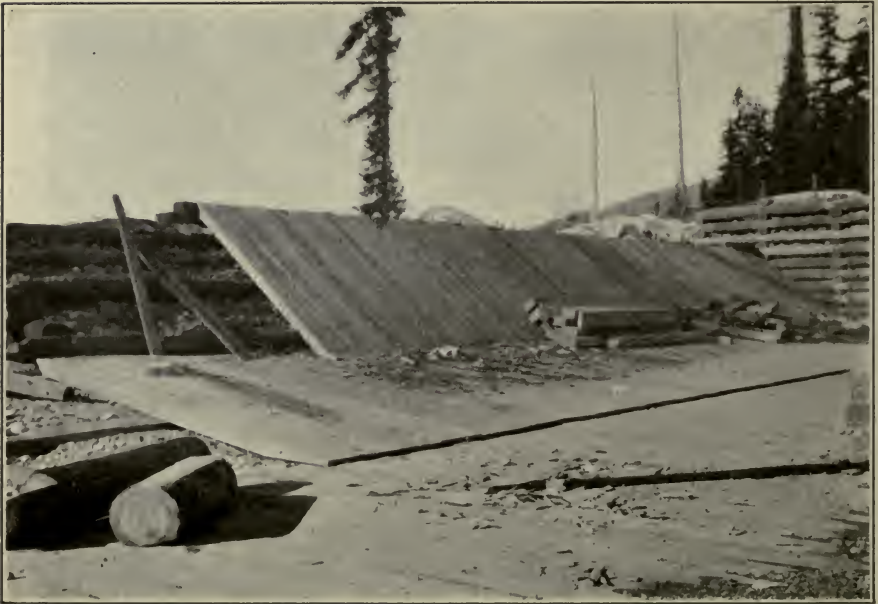
FIG. D.—Apron of partly finished timber dam. Yakima Project, Wash.
