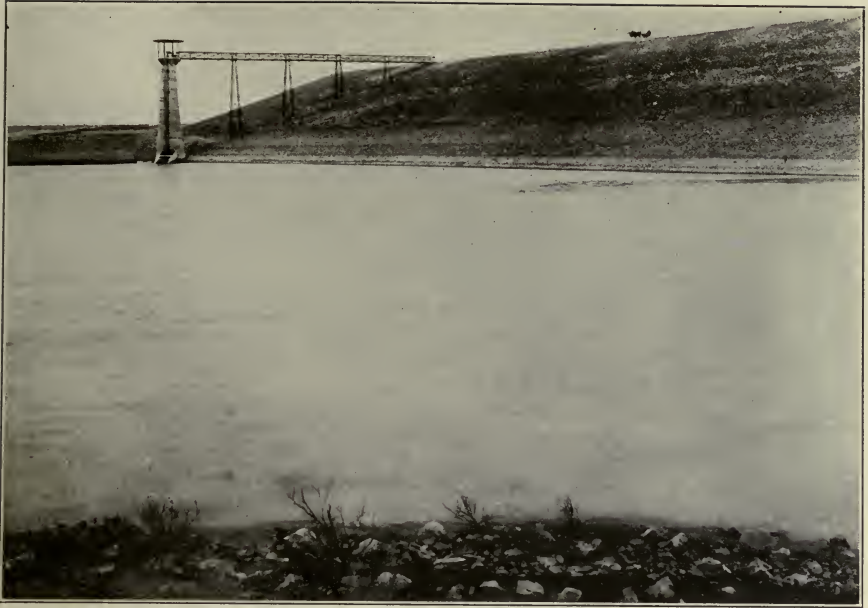
FIG. A.—Gate tower and bridge from earth dam, forming Cold Springs Reservoir. Umatilla Project, Ore.
