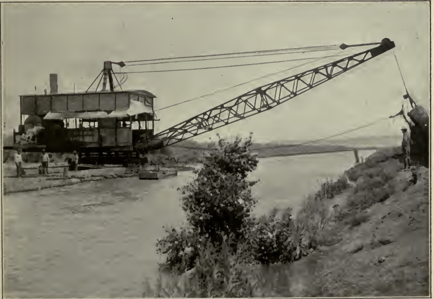
FIG. B.—Enlarging canal by use of excavator with drag-line working from one side of canal. Salt River Project, Ariz.
