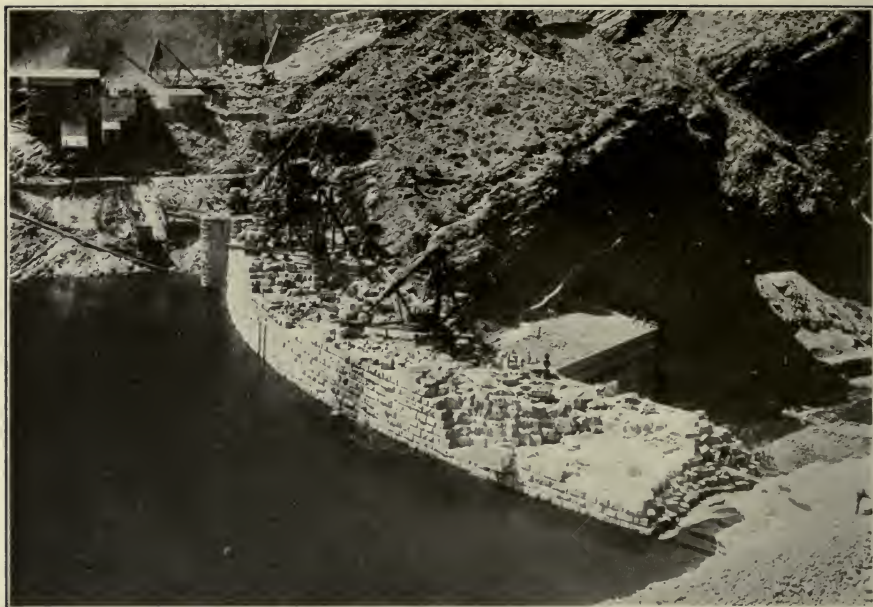
FIG. C.—Rubble masonry dam; lower portion of Roosevelt Dam, Ariz. (See finished dam, Plate XI, Fig. D.)
