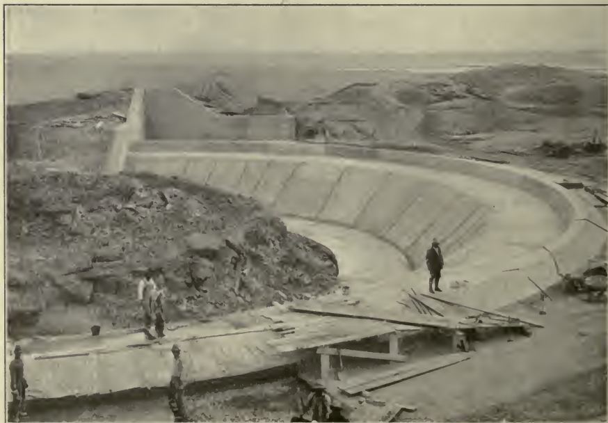
FIG. D.—Spillway for earth dam. Belle Fourche Project, So. Dak.
