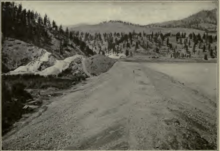
FIG. D.—Completed dam built by hydraulic process, shown above.
