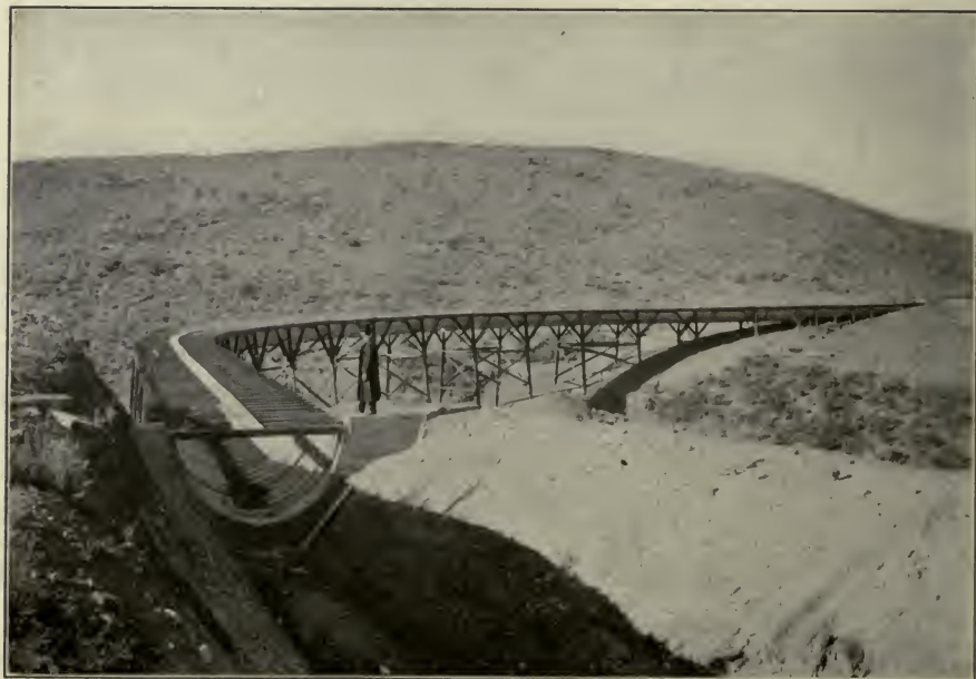
FIG. D.—Metal flume on timber trestle.
