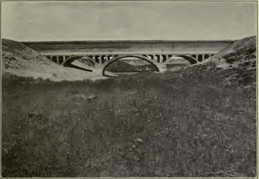
FIG. A.—Concrete flume carrying water of main canal across side drainage lines. North Platte Project, Wyo.-Nebr.
