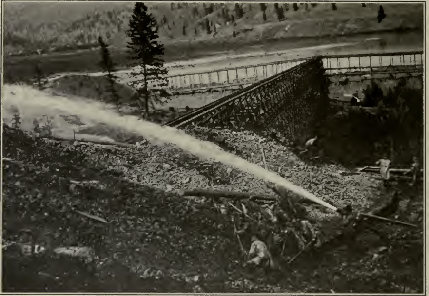
FIG. C.—Hydraulic construction of earth dam, giant in foreground washing earth and small rocks into flumes supported on trestles and conveying materials to site of dam. Okanogan Project, Wash.
