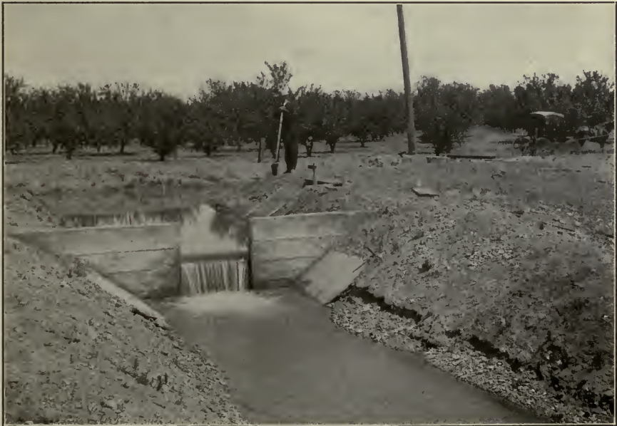
FIG. B.—Concrete box and drop on distributory in place of earlier form of wooden construction. Orland Project, Cal.
