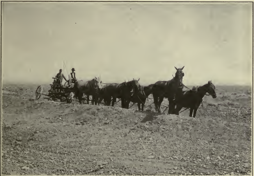
FIG. B.—Throwing up small laterals by means of four-horse road machine. Huntley Project, Mont.
