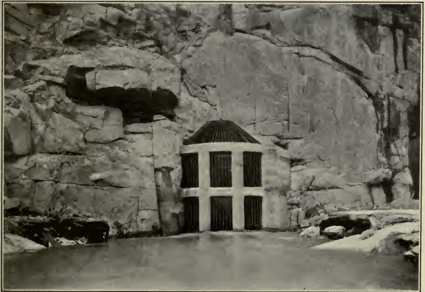
FIG. B.—Grillage protecting entrance to gates. Pathfinder Reservoir. North Platte Project, Wyo.
