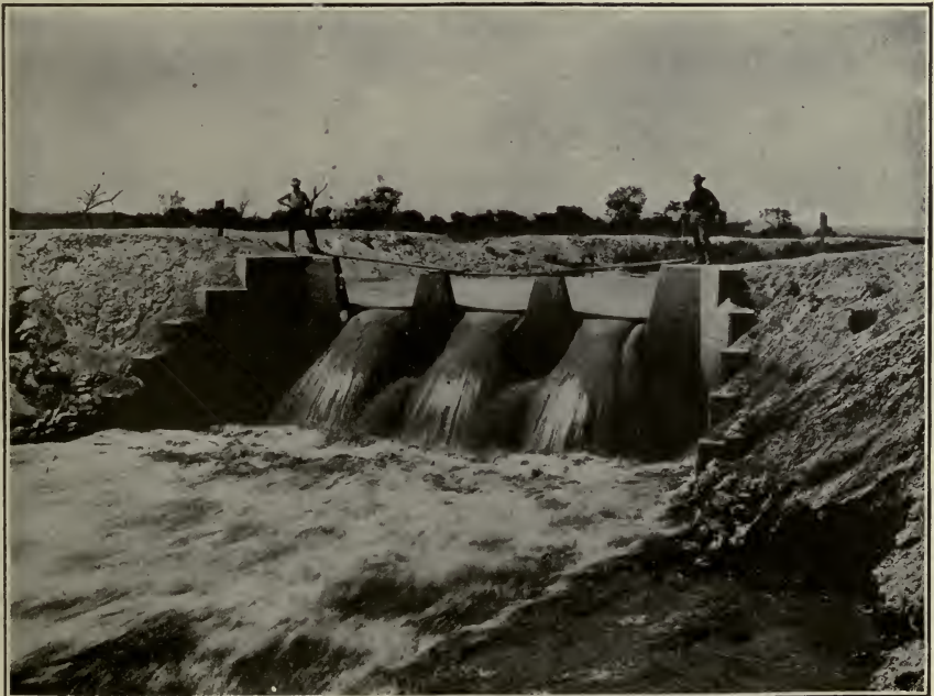
FIG. B.—Notched check and drop with projecting lip beneath each notch to diffuse and break the force of the falling water. Rio Grande Project, N. Mex.
