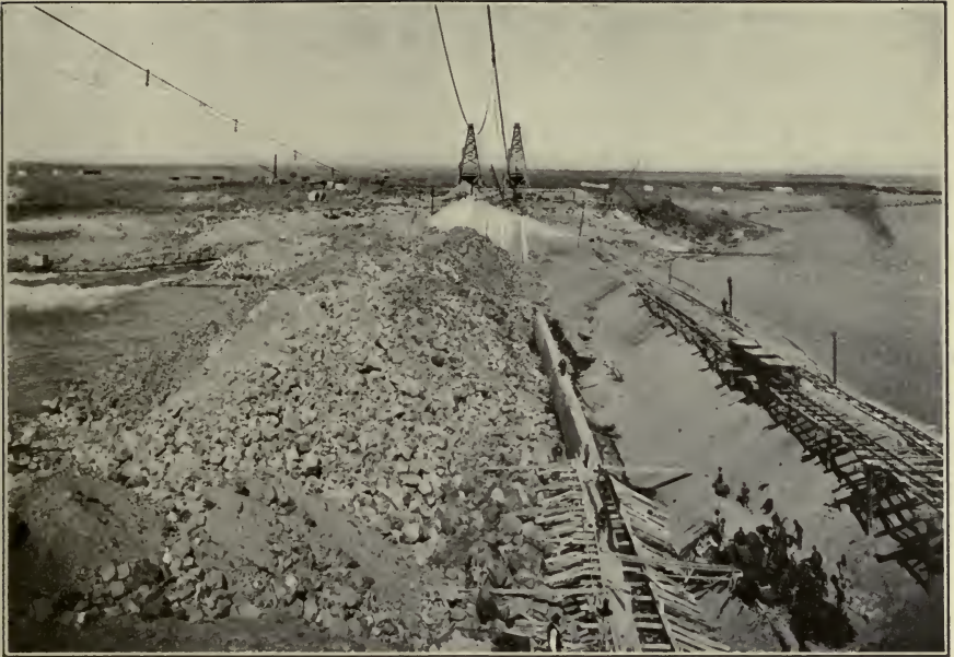
FIG. A.—Earth and rockfill dam under construction, with low concrete core wall, gravel and earth is being dumped on upper side with loose rock below, Minidoka, Idaho.
