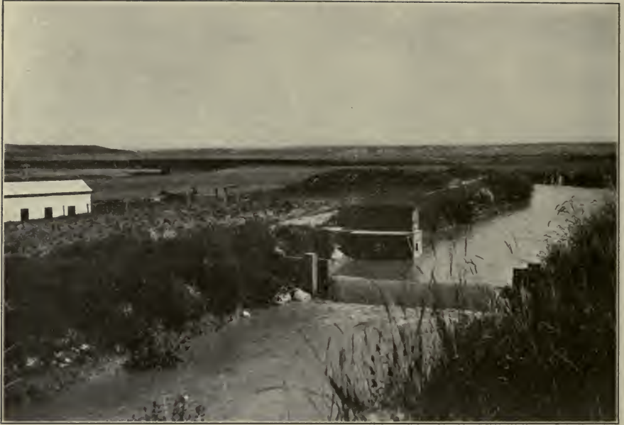
FIG. C.—Weir and self-registering gage. Williston Project, No. Dak.
