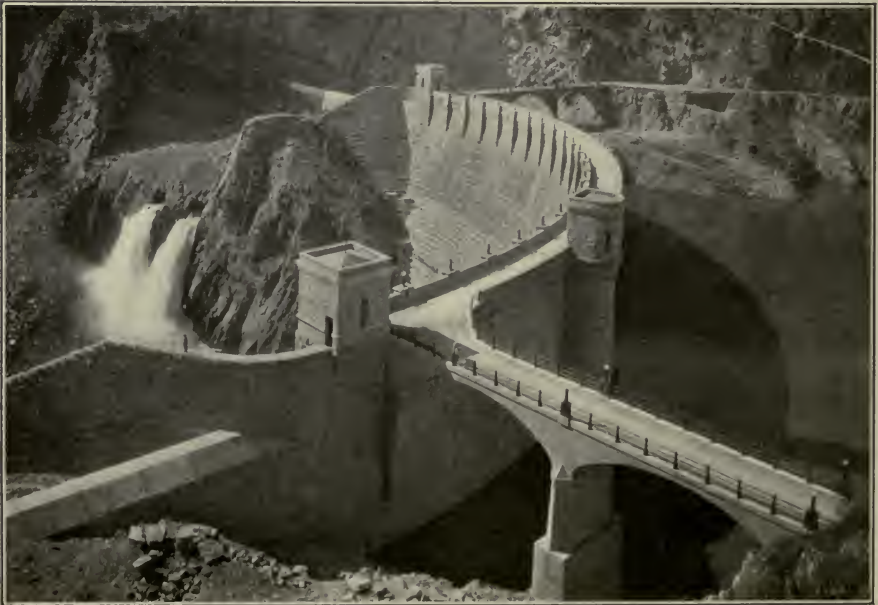
FIG. D.—Spillways of Roosevelt Dam. Salt River Project, Ariz.
