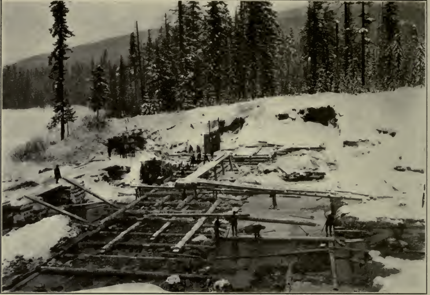
FIG. C.—Foundations for timber dam. Yakima Project, Wash.
