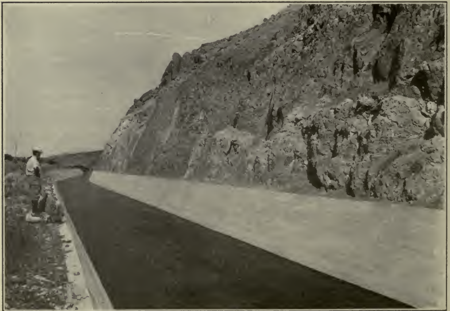
FIG. D.—Concrete lined canal in shattered rock, carrying water of Truckee River to Carson River. Truckee-Carson Project, Nev.
