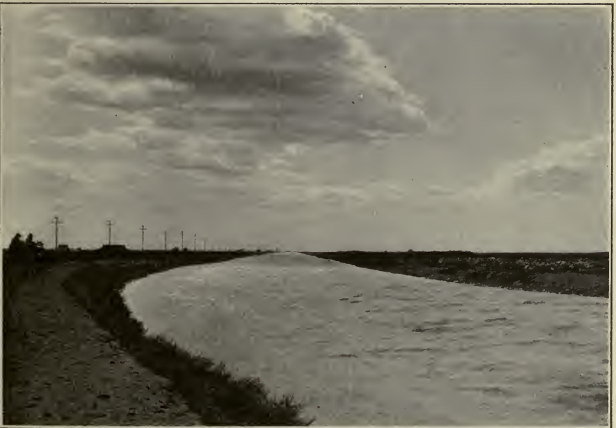
FIG. B.—Main northside canal of Minidoka Project, Idaho. Illustrative of the larger irrigation canals, with power transmission lines located on the bank.
