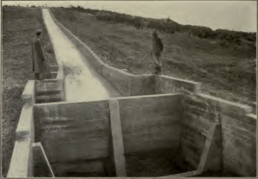
FIG. C.—Concrete chute, built instead of a series of drops, and terminating in a water cushion with concrete baffle board. Boise Project, Idaho.
