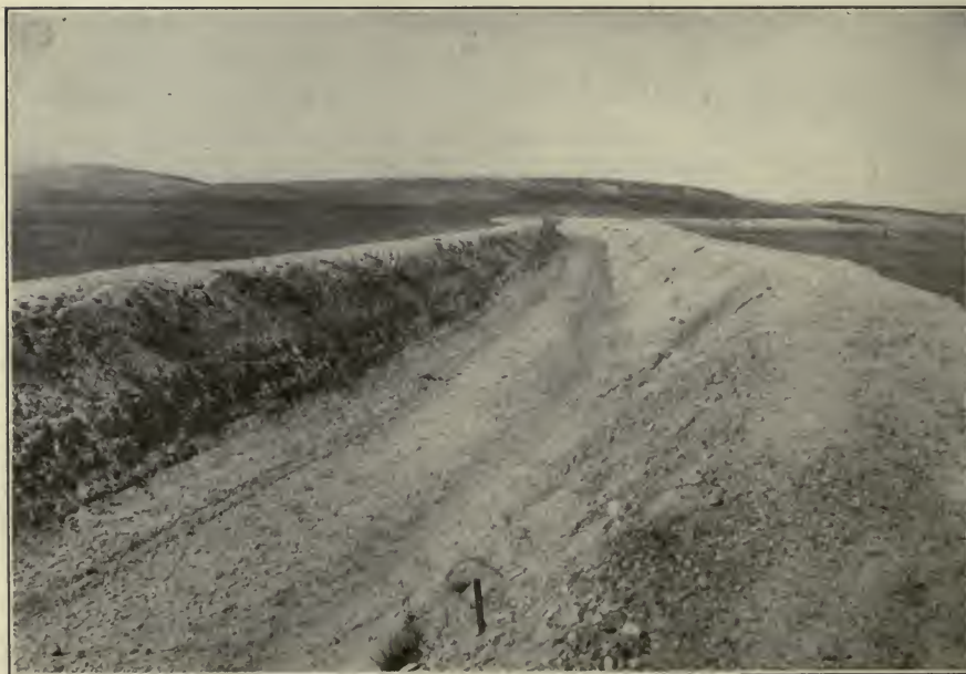
FIG. D.—Finished canal with both upper and lower banks. Lower Yellowstone Project, Mont.
