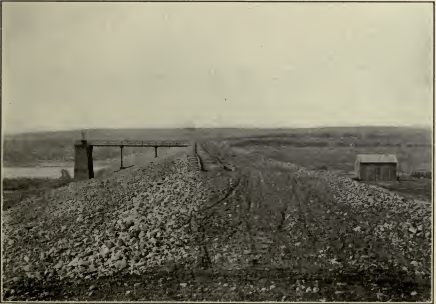
FIG. B.—Earth dam partly protected by heavy gravel on water side. Boise Project, Idaho.
