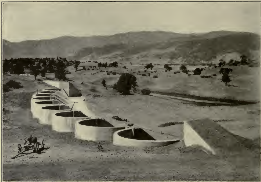
FIG. C.—Spillway with effective lengths increased by curved outlines. Orland Project, Colo.
