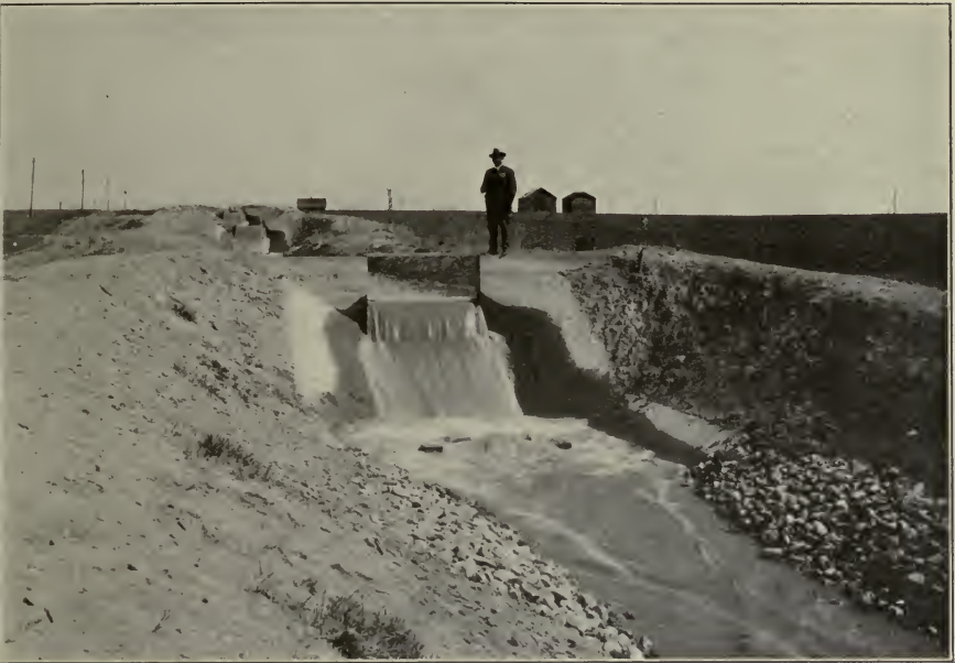
FIG. A.—Series of checks and drops with inclined chutes terminating in water cushion with concrete blocks to break the force of the water. North Platte Project, Nebr.
