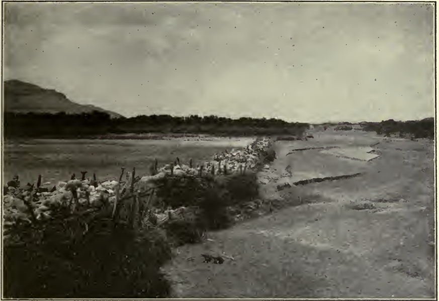
FIG. A.—Brush and stone dam, typical of pioneer conditions. Las Cruces canal, Rio Grande, N. Mex.
