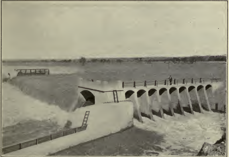
FIG. B.—Concrete headworks with steel gates. Interstate canal, North Platte Project, Nebr.
