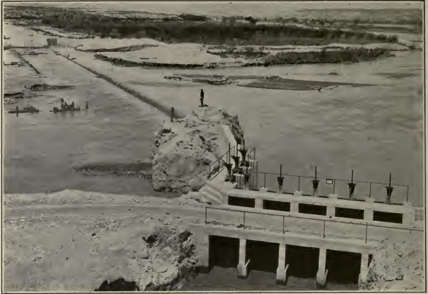
FIG. C.—Concrete headworks and roadway, Mesilla Valley canal. Rio Grande Project, N. Mex.
