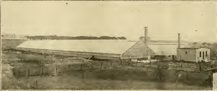
Garland Trussed Iron Frame House 43x300, Built for Dobbs &amp; Sons, Auburn, N. Y.
