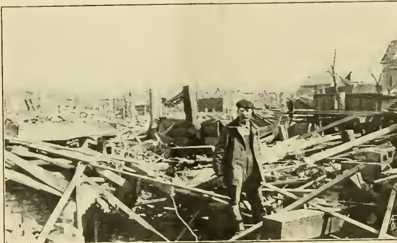
HANS JENSEN AND HIS DEMOLISHED GREENHOUSES.
