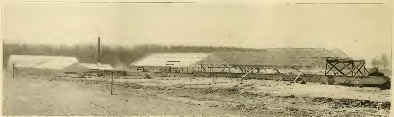
GENERAL VIEW OF UNCOMPLETED RANGE AT ILLINOIS EXPERIMENT STATION.
