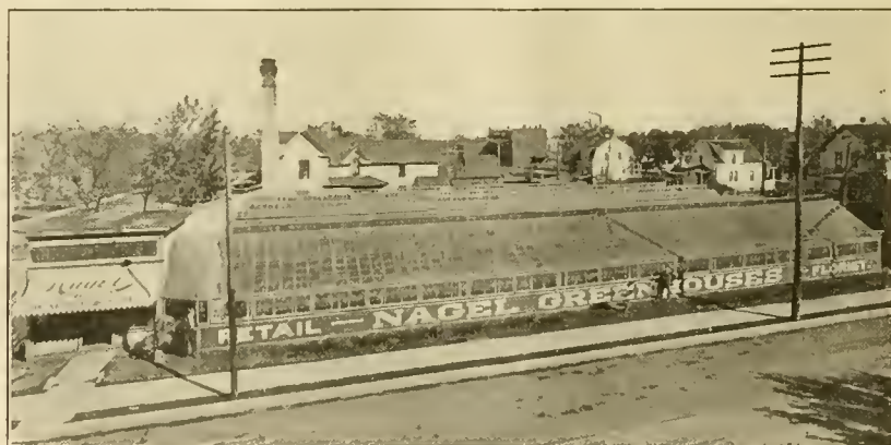
E. NAGEL & CO.'S GREENHOUSES, MINNEAPOLIS, MINN.
