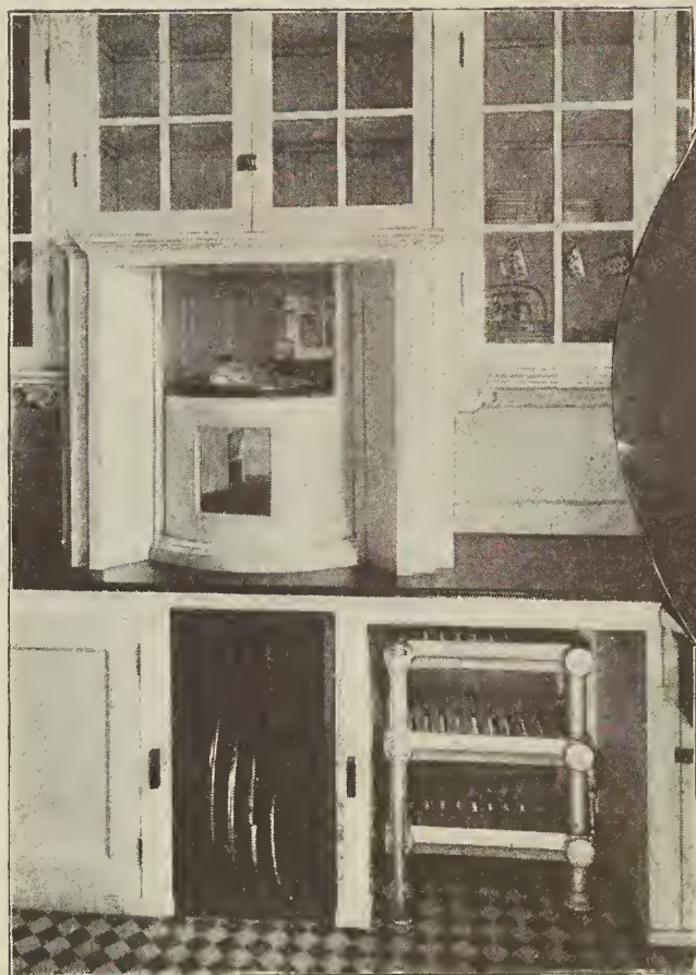
In this pantry closet, dishes are passed through the revolving center from the kitchen. Below are a tray compartment and a warming-closet
