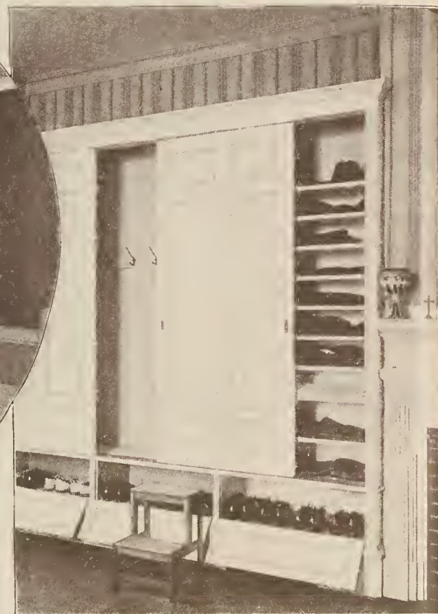
This closet, the depth of the mantel, has plenty of hanging-space and shelves for hats and clothing, with shoe-closets below
