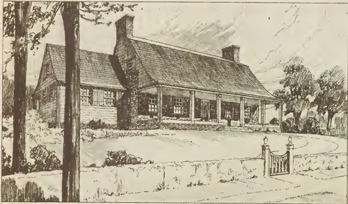
THIS MODERN ADAPTATION LENDS ITSELF TO ECONOMY, USE OF LOCAL MATERIALS AND CHARMING DECORATIVE TREATMENT
