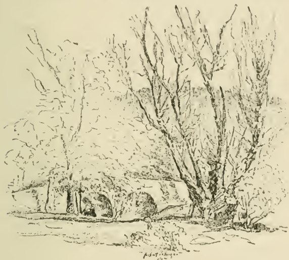
Rex Avenue Bridge
