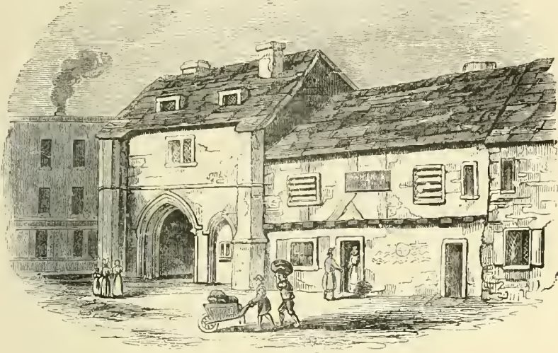
Bermondsey.—Remains of the Conventual Buildings.
