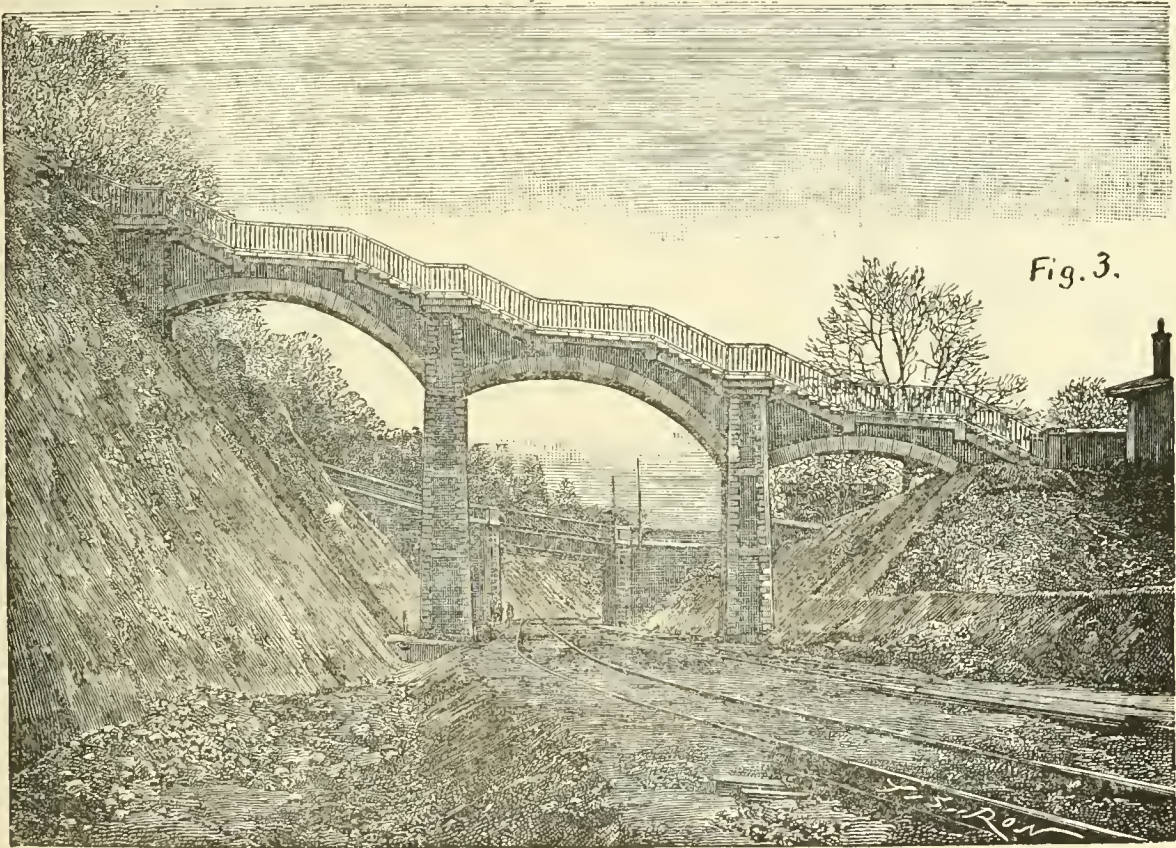
ROAD-CROSSING BRIDGE, BAS MEUDON, FRANCE.
