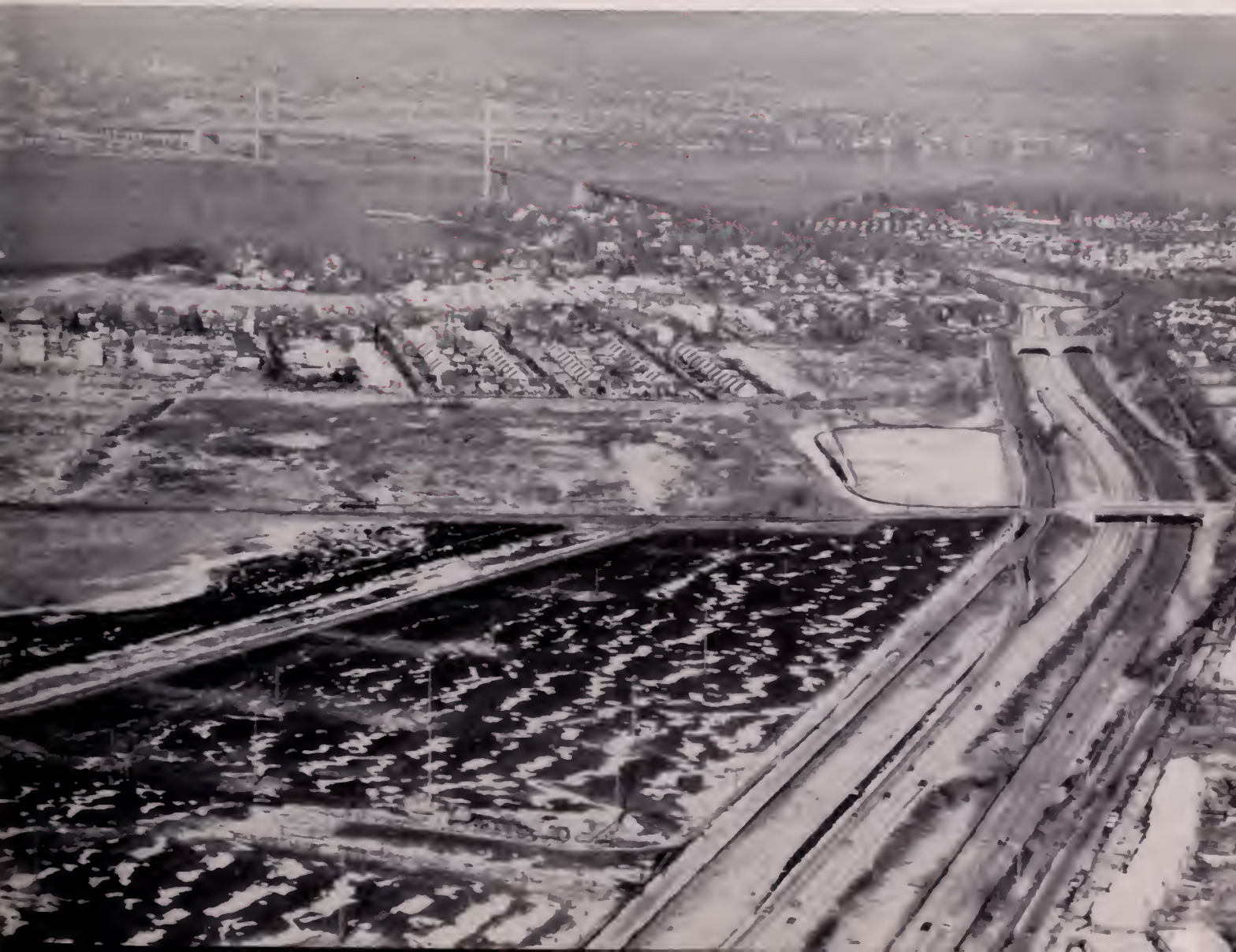
WHITESTONE EXPRESSWAY LOOKING NORTHWARD — BRONX WHITESTONE BRIDGE IN BACKGROUND
