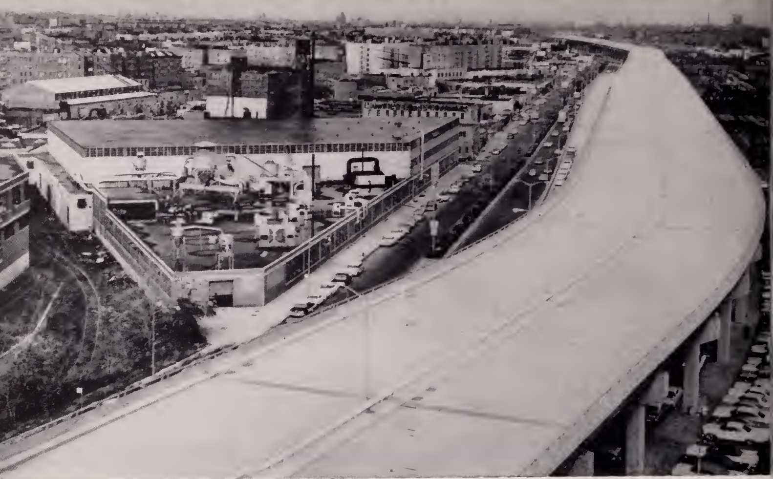
ELEVATED SECTION OF BRUCKNER BOULEVARD LOOKING NORTH — BRONX
