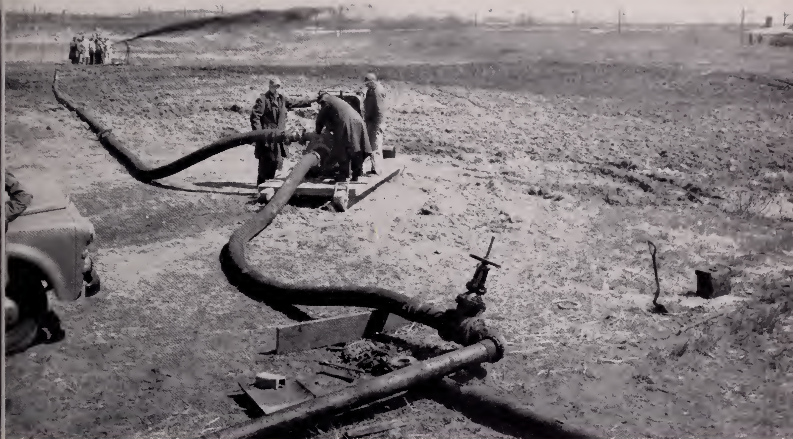
DREDGING OPERATIONS AT MARINE PARK — BROOKLYN
