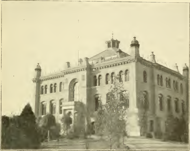
FIG. 3.—MAIN BUILDING, DIVISION I.
