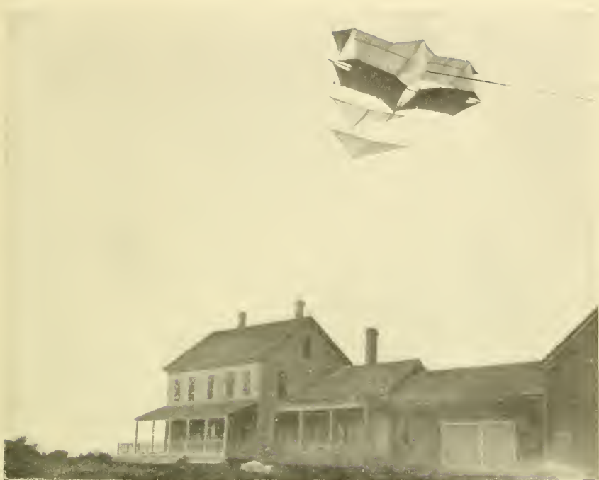
FIG. 3.—LAMSON'S AERO-CURVE KITE.
