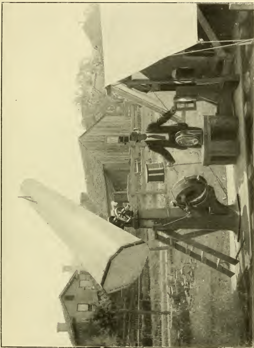
CELOSTAT WITH EQUATORIAL CAMERA AND SHOWING THE GREAT LENS AND PRISM.
