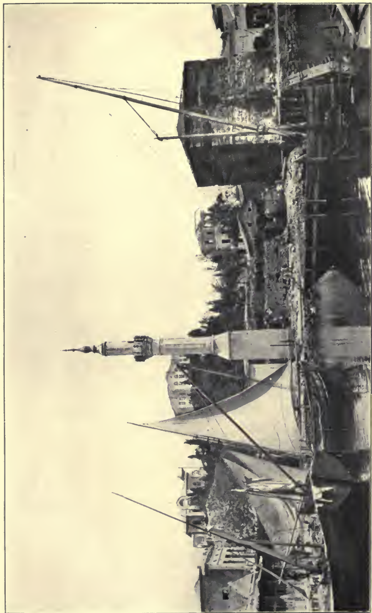
The smashed mosque by the waterfront after the bombardment of the town of Gallipoli.
