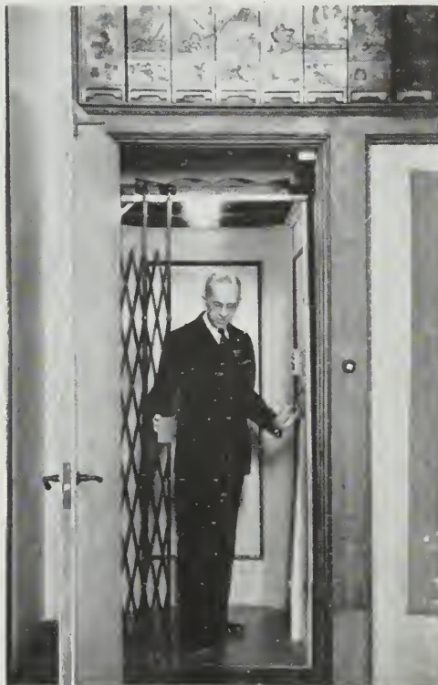
"Elevette" (in shaft)
