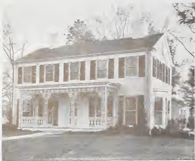
Combination of Smyser-Royer Cast Iron Veranda Designs on Residence of Claude Beene, Esq., Shreveport, La. Edw. Niels, Architect.
