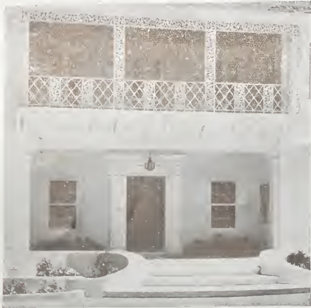
Smyser-Royer Company Cast Iron Veranda Design No. 75 a. used by Atlee B. and Robert M. Ayres, Architects, San Antonio, Texas
