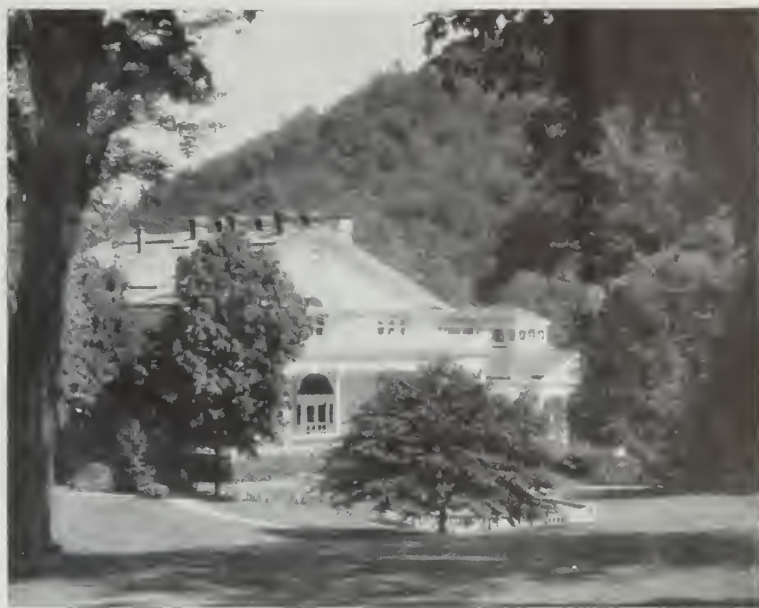
The Bath House, heart of The Homestead's Spa, seen from a neighboring hillside
