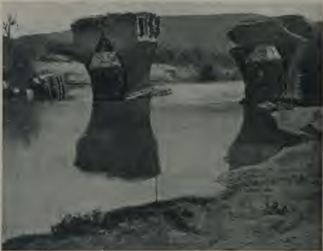
FIG. 15. AESEPUS BRIDGE. VIEW FROM NORTH.
