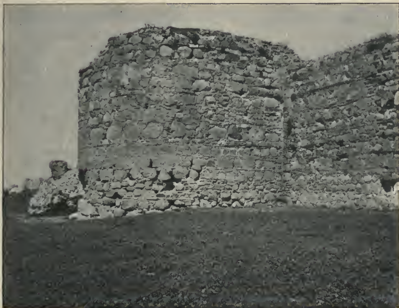
FIG. 6. ULUBAD: TOWER ON THE SOUTH WALL.
