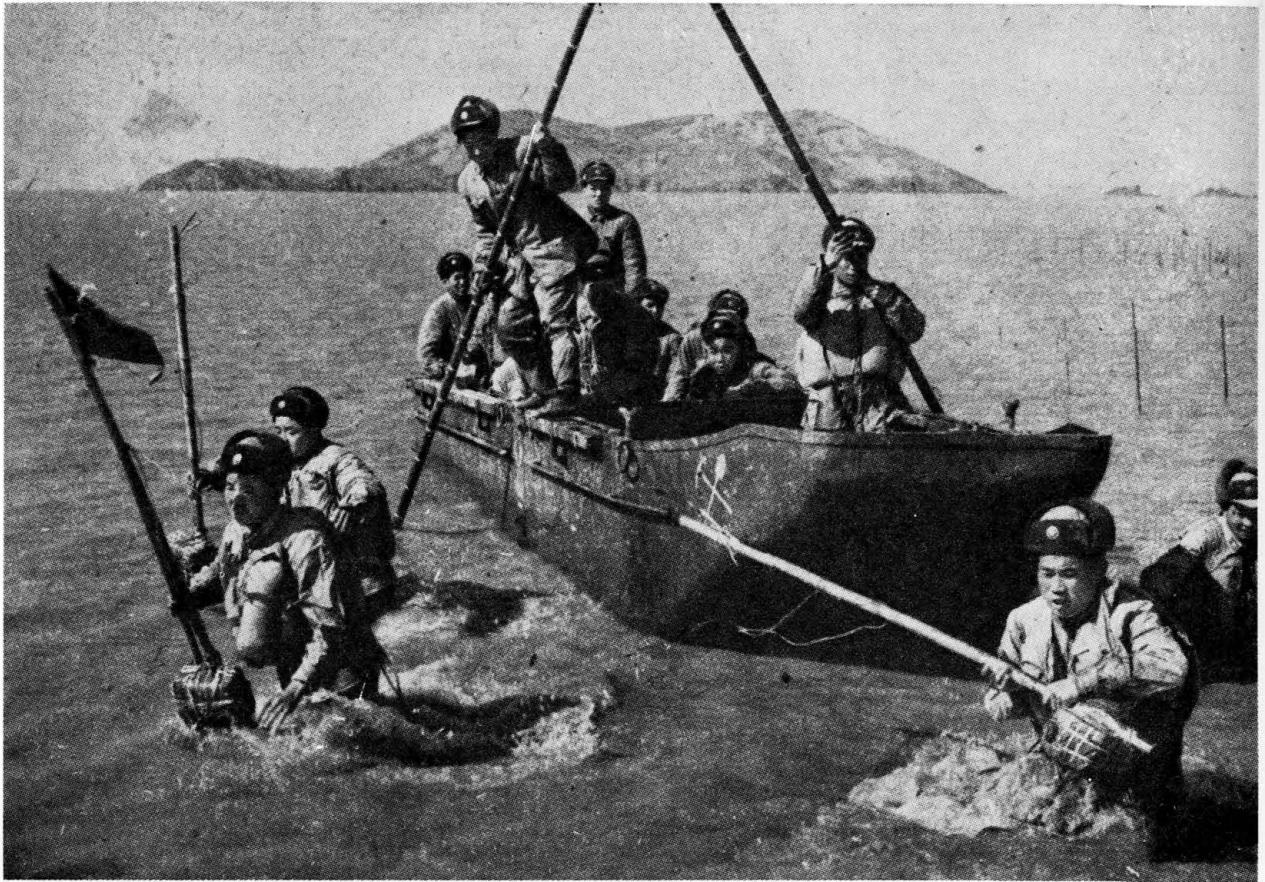
Figure 122. Steel Ponton Boat with Engineer Demolition Team.
